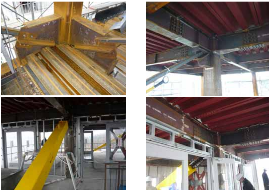
Figure 8. Interior views of the building specimen under construction (Dec. 2008 and Jan. 2009)
