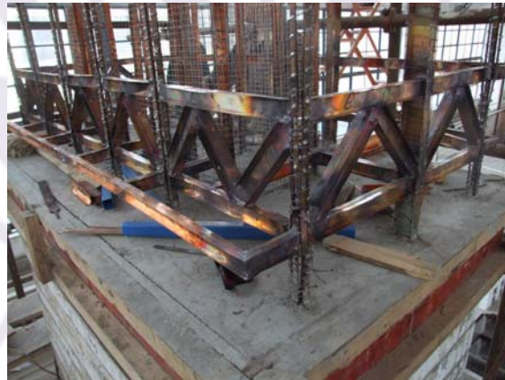
Belt Truss Storey
