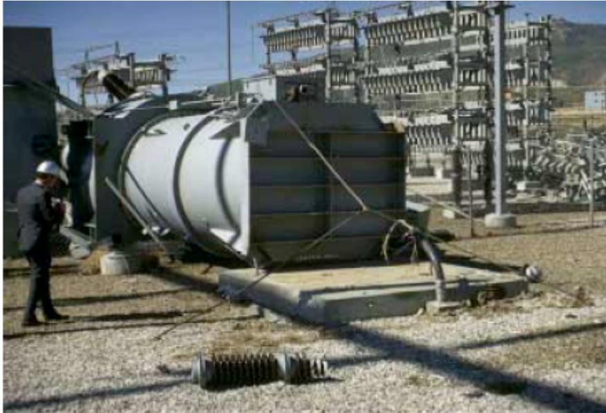
Figure 1.1. Overturned electrical equipment at Sylmar Converter Station damaged during the 1971 San Fernando earthquake (top), and a detail showing the failed back-left restrainer (bottom). Photos taken from the Steinbrugge collection, NISEE, University of California, Berkeley.
