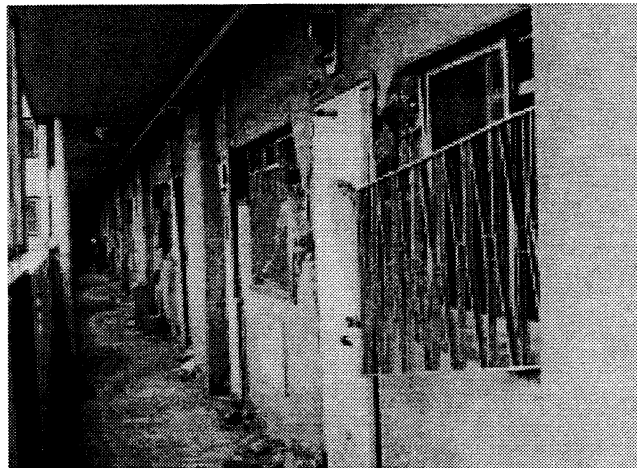
Fig. 6: Damage of non-structural elements
