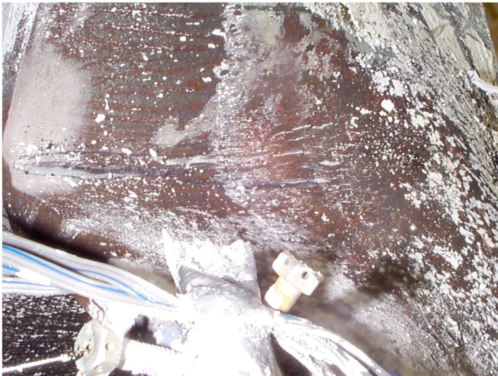
Figure 5-51 Ductile tears in the beam top flange of RC06
