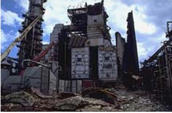
**Figure 4-28. Damage to heater unit caused by collapse of heater stack**
