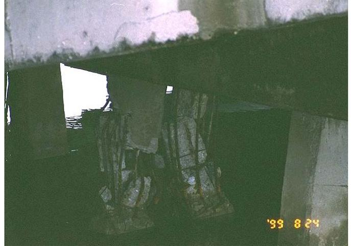
**Figure 4-35. Failure of battered reinforced concrete piles beneath jetty, Petkim facility**
