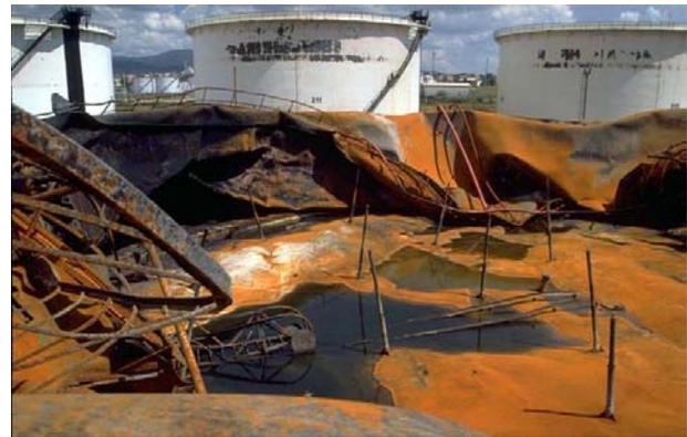
**Figure 4-25. Destroyed walls, walkways and floating roof of tank in Figure 4-24**
