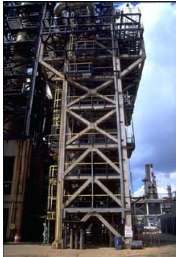
**Figure 4-30b. Undamaged reinforced concrete framing, Tupras refinery**
