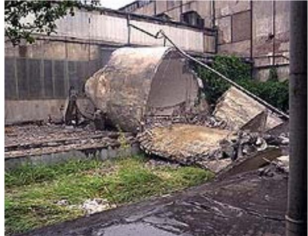
Figure 4-62b. Collapsed silo, SEKA paper mill
