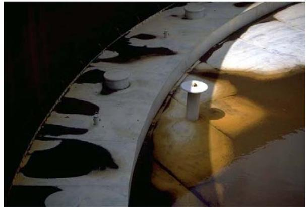
**Figure 4-17. Perimeter seal of floating roof in Tank 211**
