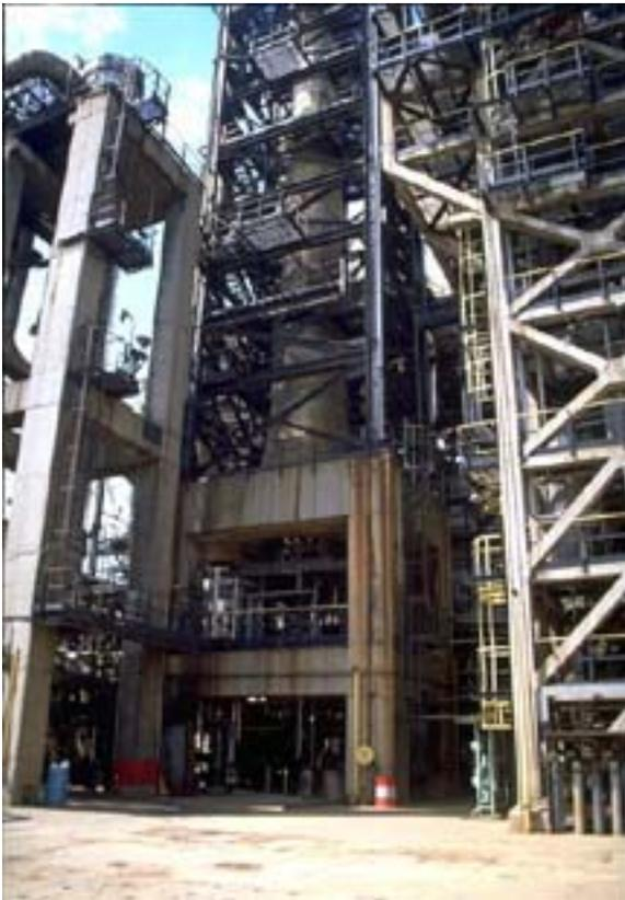
**Figure 4-30a. Undamaged steel-braced framing, Tupras refinery**
