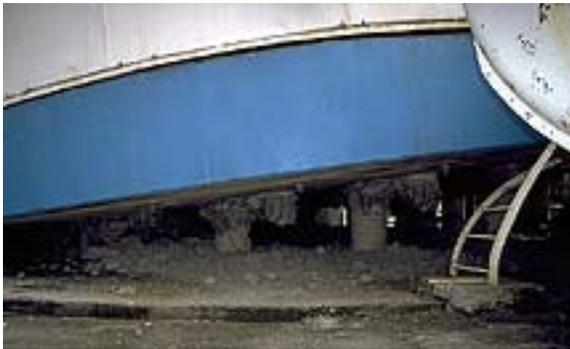
**Figure 4-59a. Failed columns beneath slab under liquid oxygen tank, Habas facility**
