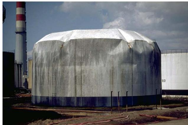
**Figure 4-26. Gross expansion of fixed roof tank adjacent to tank of Figure 4-24**
