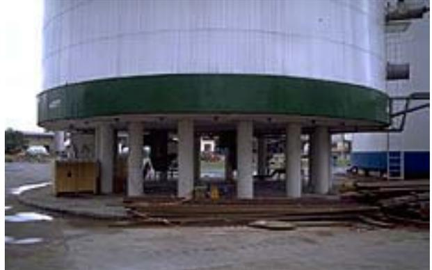
**Figure 4-56. View of Reinforced concrete framing at base of undamaged tank, Habas plant**
