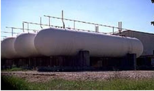
**Figure 4-63a. Typical support arrangement for cylindrical liquid gas tanks**
