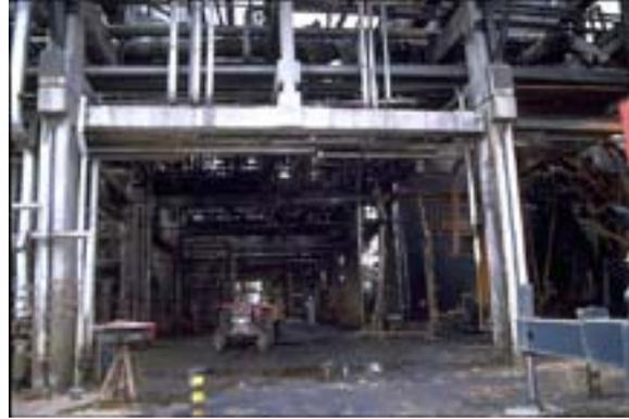
**Figure 4-29. Damage to pipework caused by collapse of heater unit**
