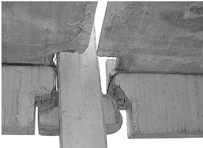
Figure 4-4 Typical plank roof construction and damaged doveled connections
