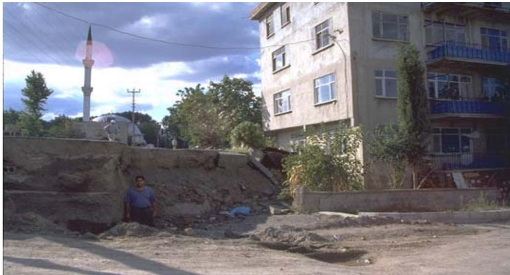
**Figure 1-2 Vertical offset near Ford Plant in Golcuk**
