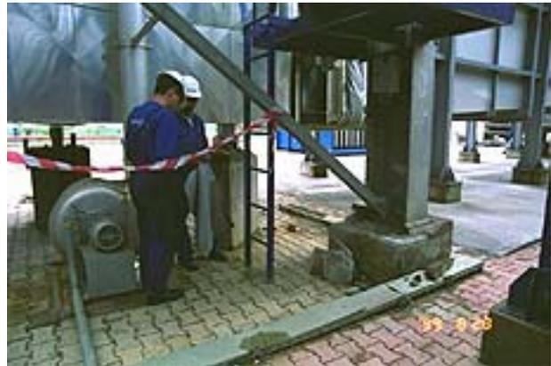
**Figure 4-47b. Damaged baseplate connection, EnerjiSA in-service steam generator**
