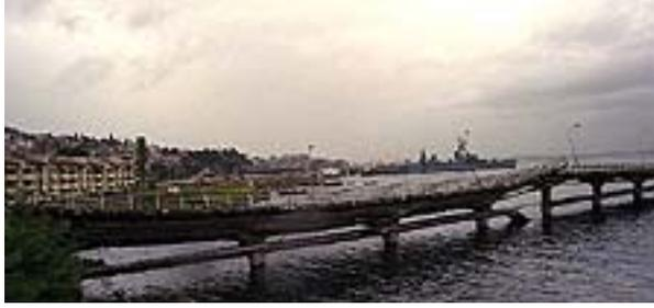
Figure 4-61a. Failure of hammerhead reinforced concrete jetty piers, SEKA paper mill
