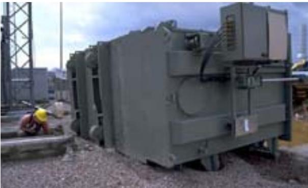
**Figure 4-45. Topped transformer in EnerjiSA transformer yard**
