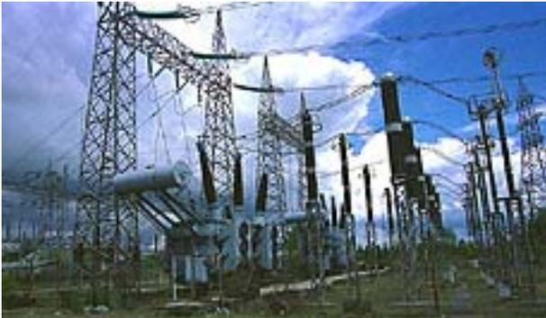
**Figure 5-53a. Elevated support frames and power transformers, Adapazari substation**
