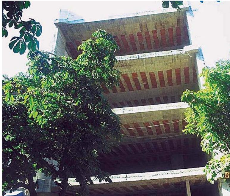
**Figure 3-11 Asmolen floor system in a four-story building**
