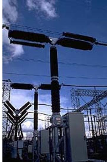
**Figure 4-51b. New T-shaped circuit breakers**
