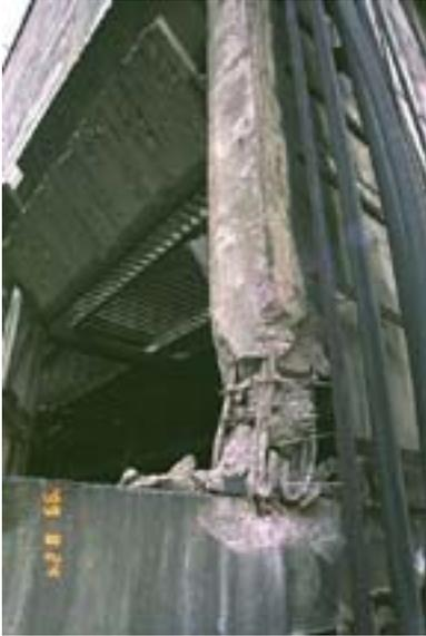
**Figure 4-33. Rebar details and damage in reinforced concrete cooling tower at Petkim**
