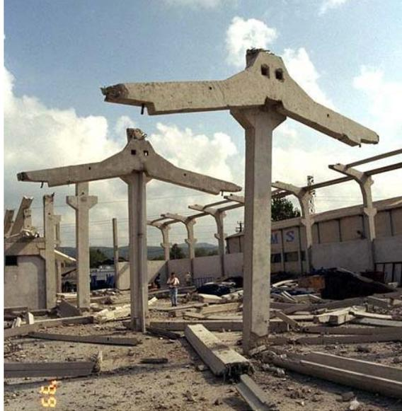
**a. failed central columns and T-shaped units**
