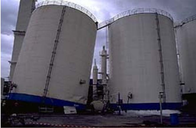
**Figure 4-57. Collapse of liquid oxygen tanks**
