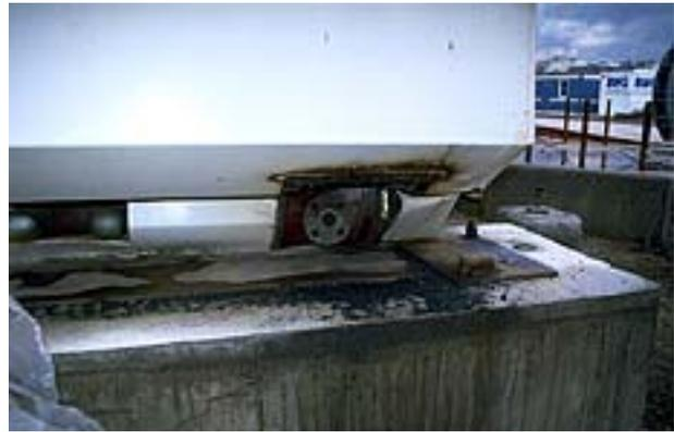
**Figure 4-46b. Failed fillet-weld connection of boiler framing to baseplate**
