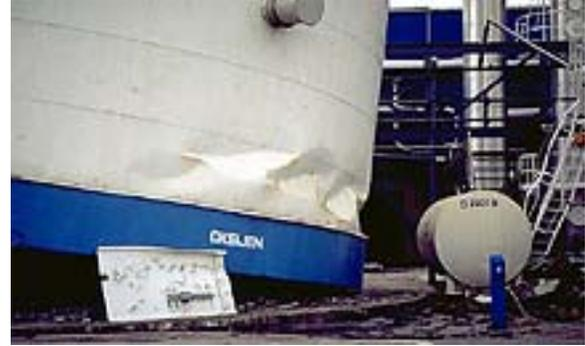
**Figure 4-58. Buckling of the outer stainless steel shell in liquid oxygen tank**
