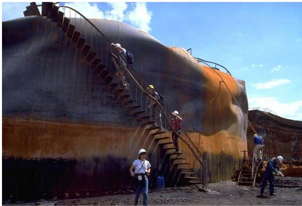
**Figure 4-24. Tank destroyed by fire in burn zone**
