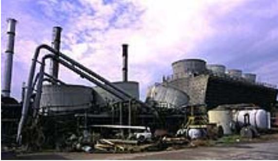
Figure 4-31. Collapsed wooden cooling tower at the Petkim petrochemical facility
