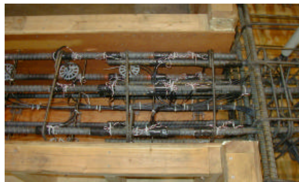
Figure 5(b) Photos of Reinforcing Cages
