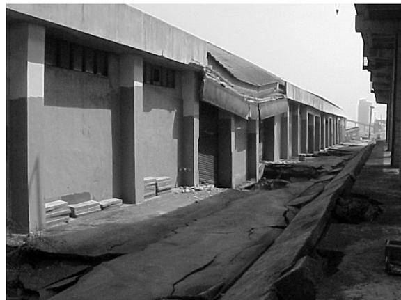
**Fig. 2.38 Structural failure due to liquefaction-induced settlement of isolated footing at Port of Taichung (from Collection, Earthquake Engineering Research Center, University of California, Berkeley).**
