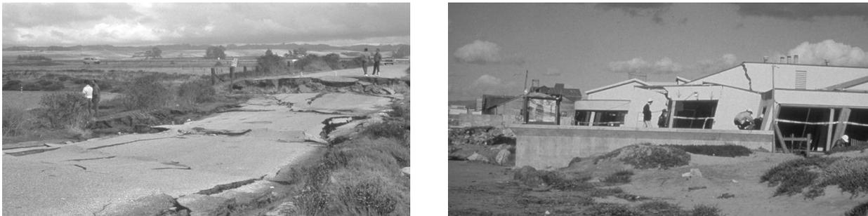
**Fig. 2.8 Lateral spreading along Sandholdt Road (left), and at Monterey Bay Aquarium Research Institute (right) at Moss Landing (courtesy of Earthquake Engineering Research Center, University of California, Berkeley).**
