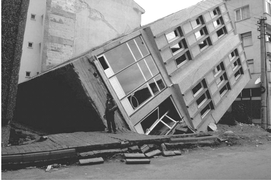
**Fig. 2.41 Liquefaction-induced bearing capacity failure in Adapazari, Turkey (from Izmit Collection, Earthquake Engineering Research Center, University of California, Berkeley).**
