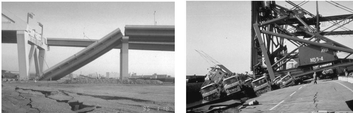
**Fig. 2.40** Examples of the effects of lateral spreading on bridges and wharf structures: (a) Nishinomiya bridge, (b) Port of Kobe wharf.
