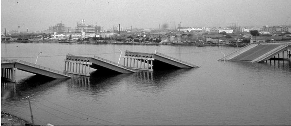
**Fig. 2.2 Failure of Showa River bridge in Niigata, Japan, due to lateral spreading.**
