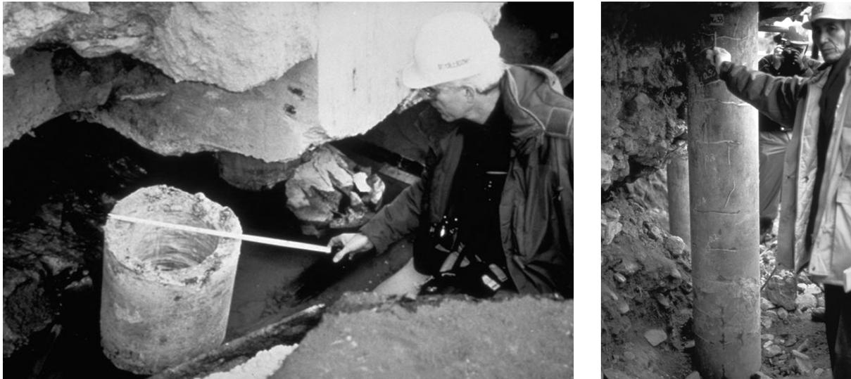
**Fig. 2.43 Pile damage due to lateral spreading in Kobe, Japan (from Izmit Collection, Earthquake Engineering Research Center, University of California, Berkeley).**
