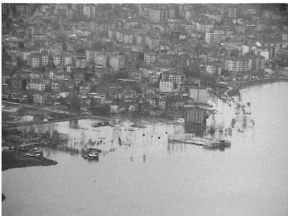
**Fig. 2.37 Coastal flooding due to liquefaction-induced subsidence in Gölcük (from Izmit Collection, Earthquake Engineering Research Center, University of California, Berkeley).**
