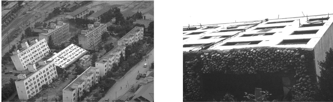
**Fig. 2.1 Kawagishi-cho apartment buildings in Niigata, Japan: (left) tilting due to bearing capacity failure; (right) close-up of shallow foundation exposed by failure.**
