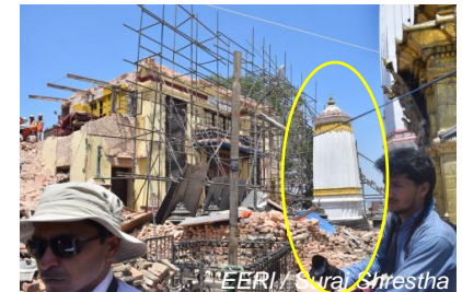
Similar Temples- Anantapur Temple (Superstructure collapsed) and Pratappur Temple (Plinth damage) of Swayambhu
