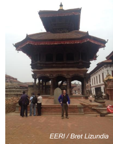
Chyasilin Mandap in Bhaktapur DS- seismically strengthened and undamaged
