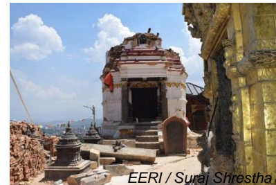
Similar Temples- Anantapur Temple (Superstructure collapsed) and Pratappur Temple (Plinth damage) of Swayambhu
