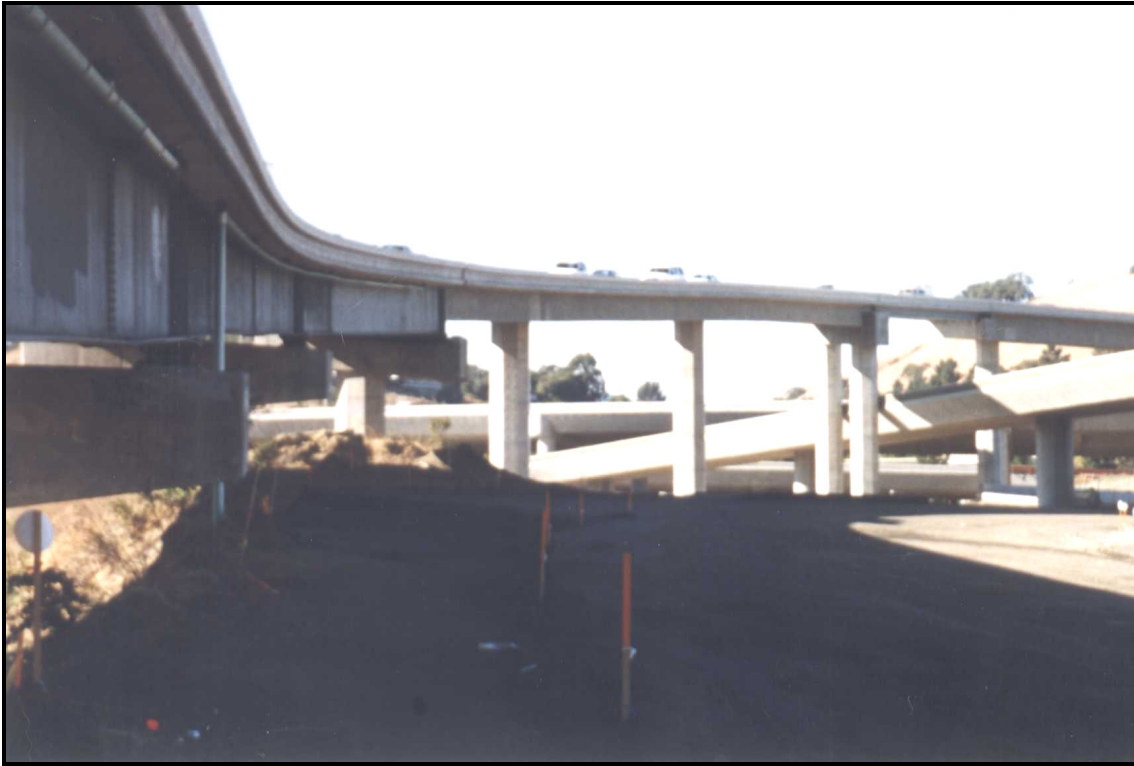
Figure 1.1 Example of a bridge structure supported on single-column extended pile shafts in the San Francisco Bay Area.
