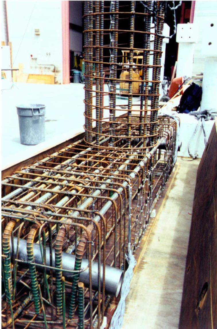
**Fig. 1.2 Beam and column joint rebar assembly**
