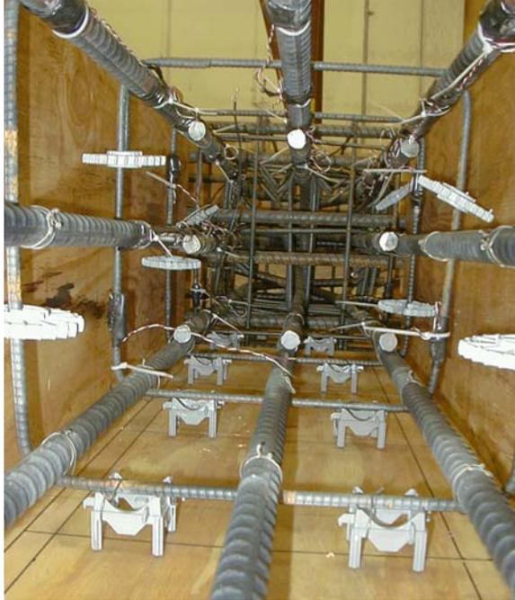
**Figure 2.8-** Column Cross Section
