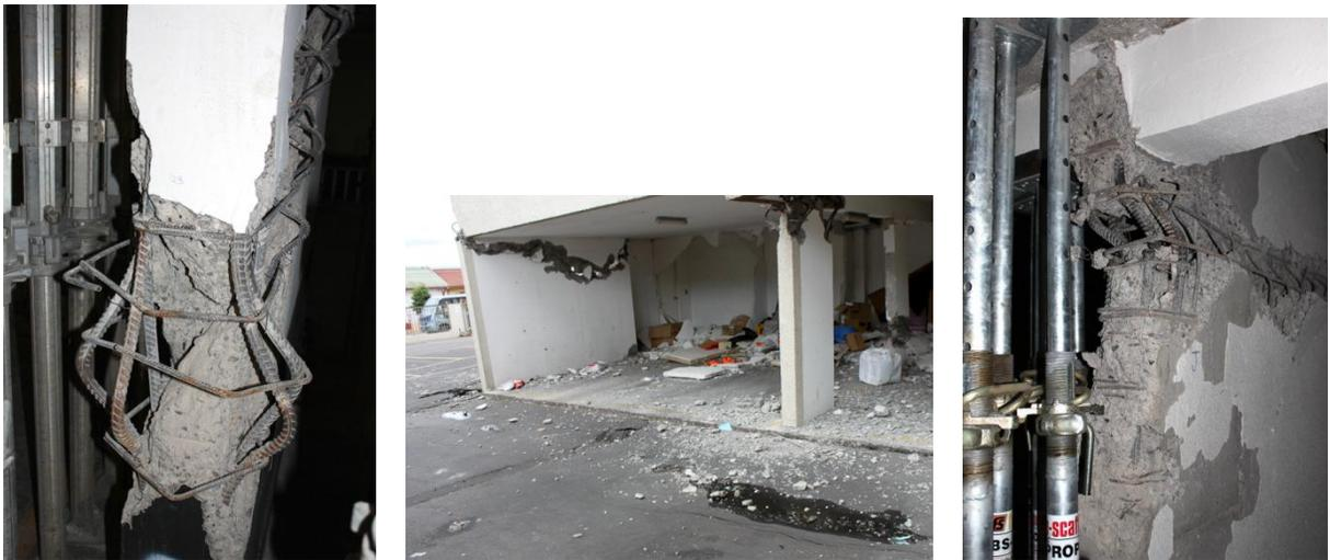
**Figure 1: Typical failure seen after February earthquake (credit: Moehle)**
