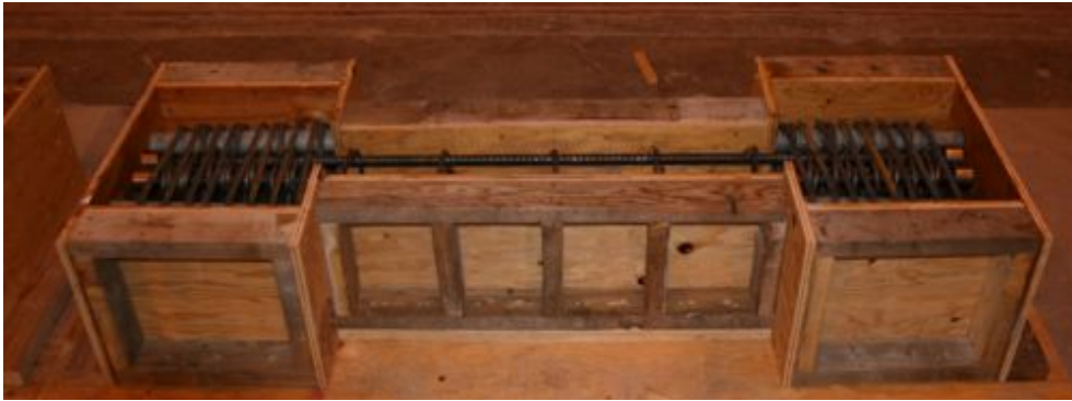
Figure 2.4: Reinforcement cage in concrete formwork
