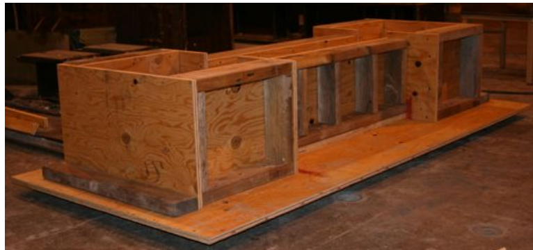
Figure 2.2: Concrete formwork
