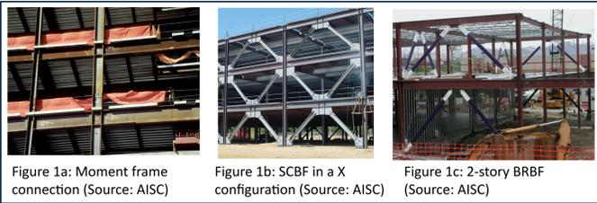
Figure 1a: Moment frame connection (Source: AISC) Figure 1b: SCBF in an X configuration (Source: AISC) Figure 1c: 2-story BRBF (Source: AISC)
