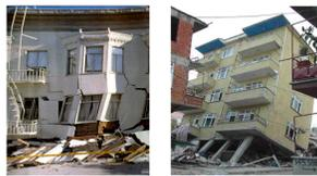
Figure 3a and 3b: The Soft-story Mechanism (Source: NISEE)
