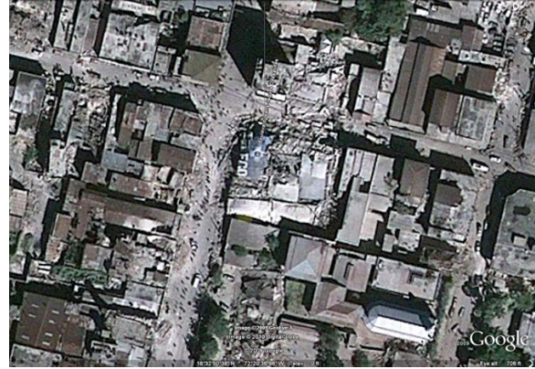
Fig. 2 Aerial view of earthquake affected intersection.
