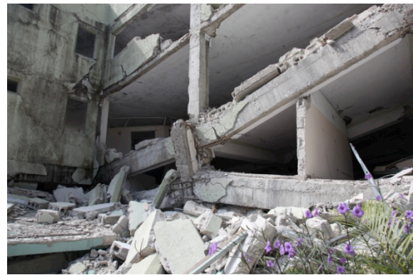
Fig. 18 Damaged Parking Lot in Haiti.
