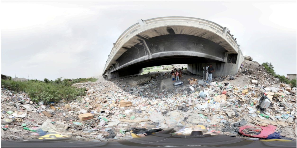
Fig. 19 Three-hundred and sixty spherical panorama of bridge.
