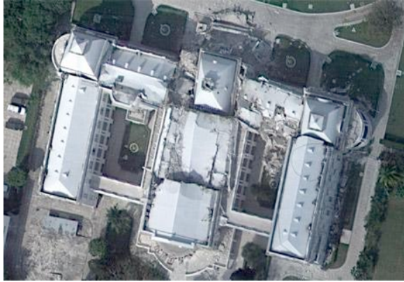
Fig. 1 Ariel view of Haiti's National Palace after the earthquake.
