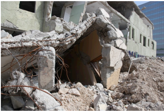
Fig. 15 Collapsed building in Haiti.
