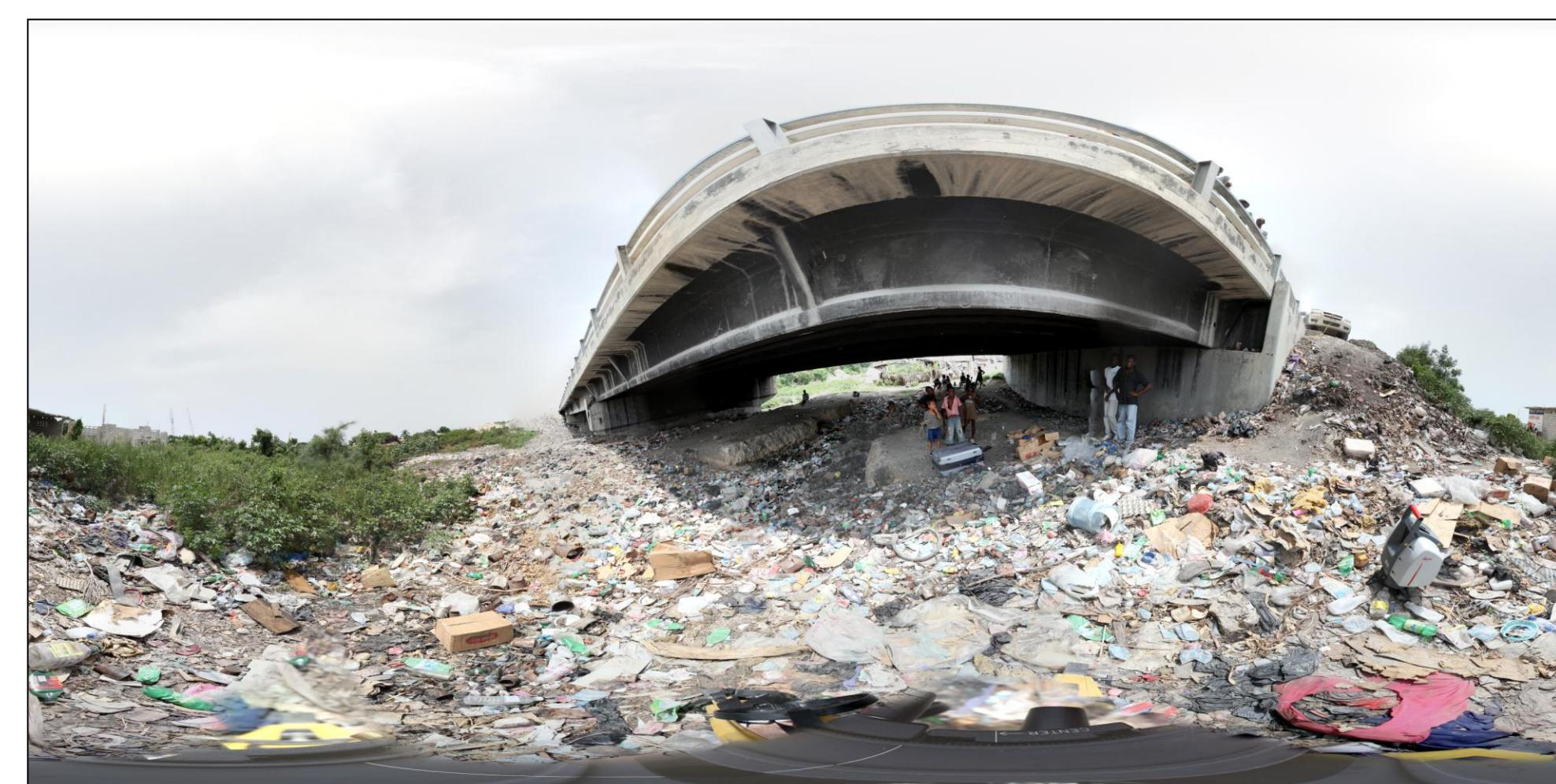
Fig. 8 Resultant three-hundred and sixty degree spherical panorama of bridge. Fisheye lens for high-definition camera was used.
