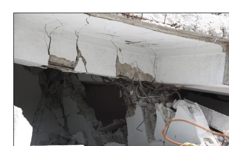
Fig. 11 Close-up of a collapsed level inside of Fig. 10.
