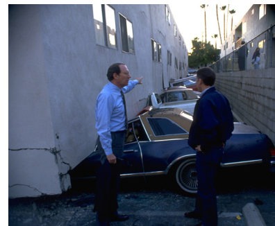
Northridge earthquake soft-story failures (source top: unknown; bottom: FEMA News Photo)
