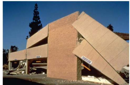
Precast parking structure at Northridge Fashion Mall after 1994 Northridge earthquake. (source: unknown)
