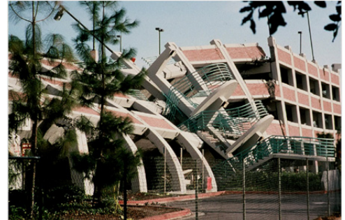
Cal State Northridge parking structure after 1994 Northridge earthquake. (source: unknown)
