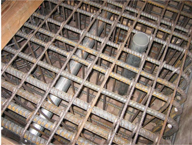
Figure 3.20: Typical Footing Reinforcement Cage
