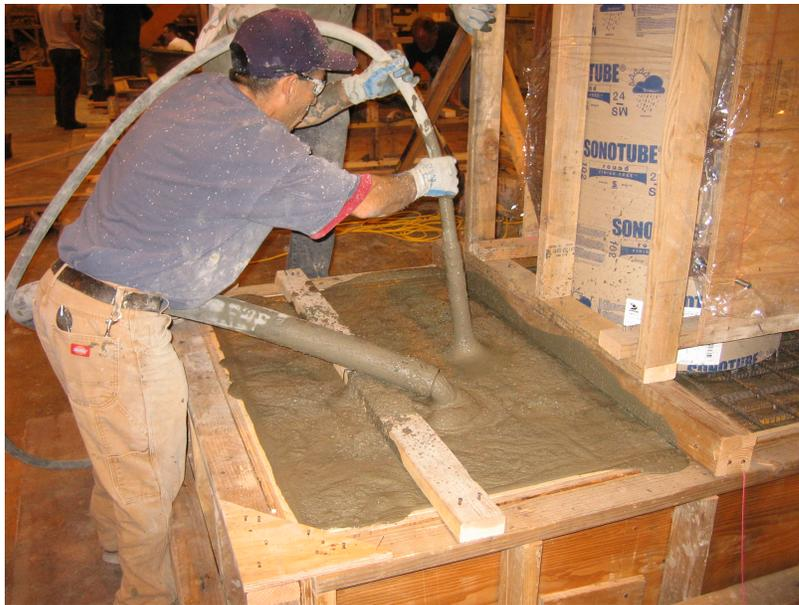
Figure 3.25: Concrete Placement and Vibration of Footing
