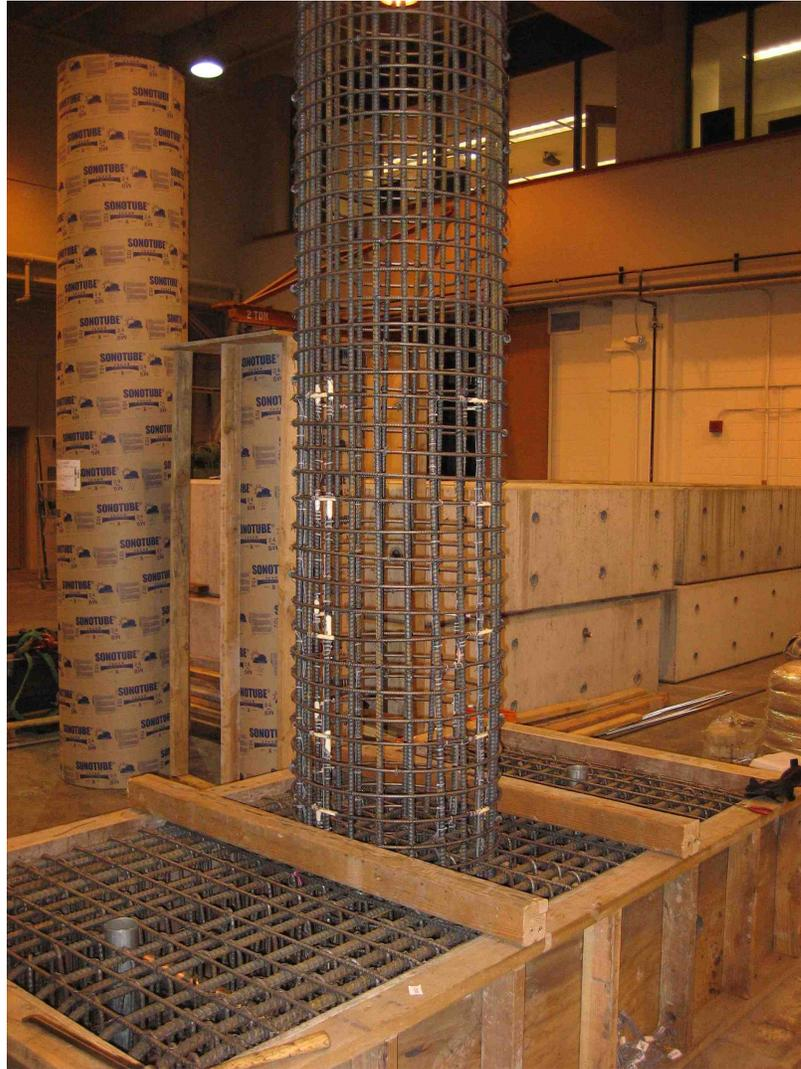
Figure 3.22: Typical Circular Column Reinforcement Cage
