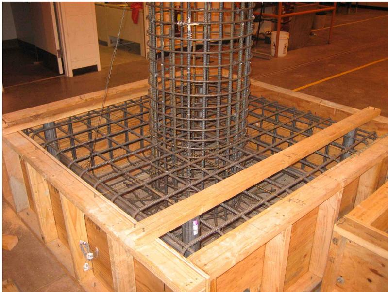
Figure 3.21: Column C4 Footing Reinforcement Cage
