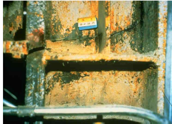
Photo provided by: Jim Malley, Degenkolb
