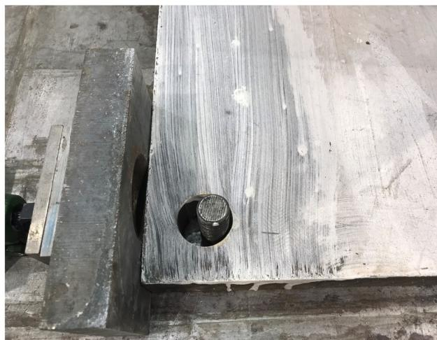
**Figure C.5** Uncentered anchor with base plate hole.
