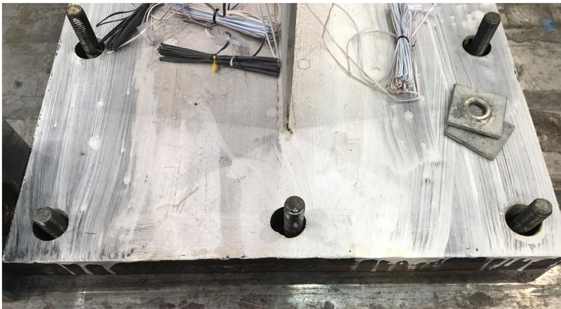
**Figure C.7** Anchors centered with base plate holes.
