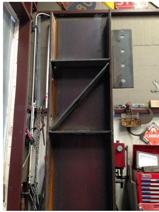
**Figure B.2** Shear tab plate and column stiffeners
