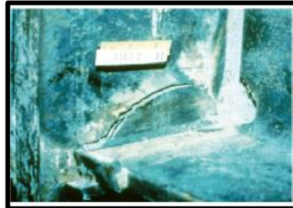
Fractures in welded steel moment frame beam-to-column connections
