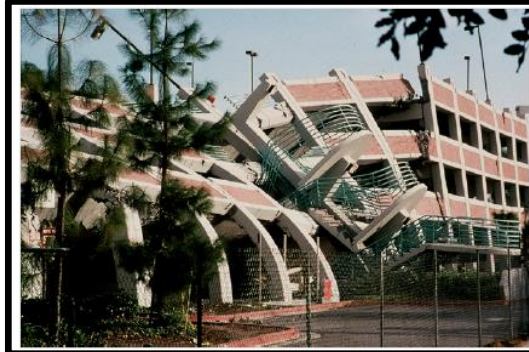
Non-ductile concrete & weak stories
