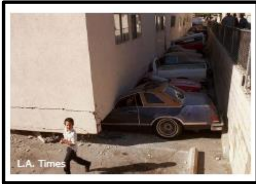
Soft & weak story wood-frame collapses
