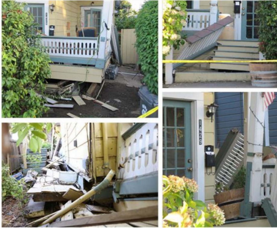
Figure 1.3 A view of a cripple wall collapse on an as-built house (top left), damage to the utility lines and gutter pipe (bottom left), and displacement as well as elevation change of the home's entrance stairs (top right) and patio railing (bottom right), 2014 Napa earthquake, Napa, California (image courtesy of Kang and Mahin [2014]).
