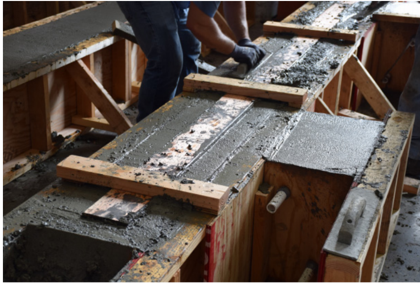
Figure 3.22 Specimen A-6 sill plate being wet set into the footing.
