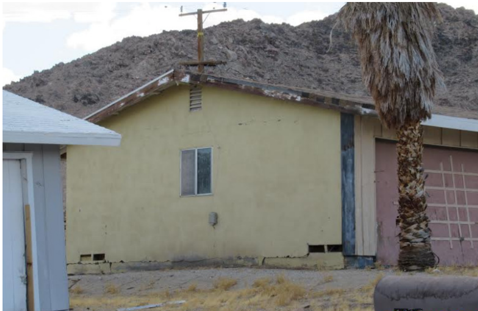
Figure 1.4 Partial foundation anchorage failure at the cripple wall of a stucco house in Trona, California (image courtesy of Cobeen [2019]), 2019 Ridgecrest earthquake, Ridgecrest, California.
