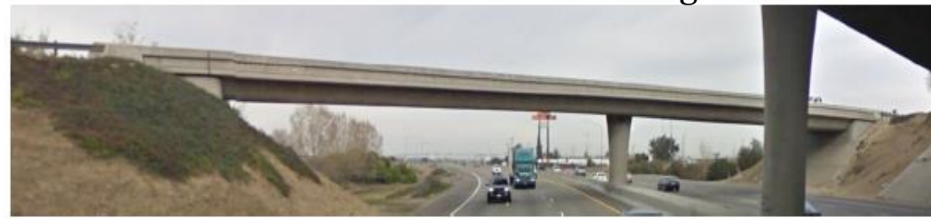
Jack Tone Road Overcrossing
