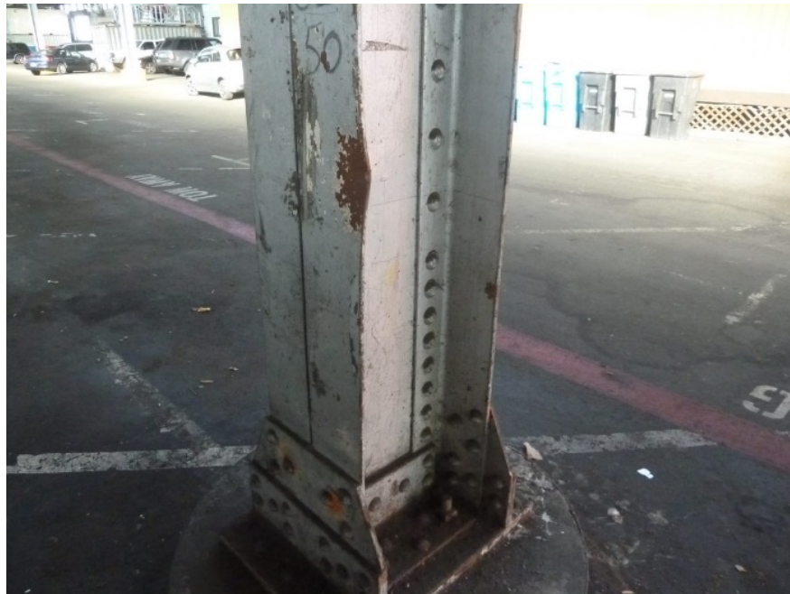
Figure 3.7: Steel columns consisted of built up sections, composed of four angle sections connected with two web plates via rivets.
