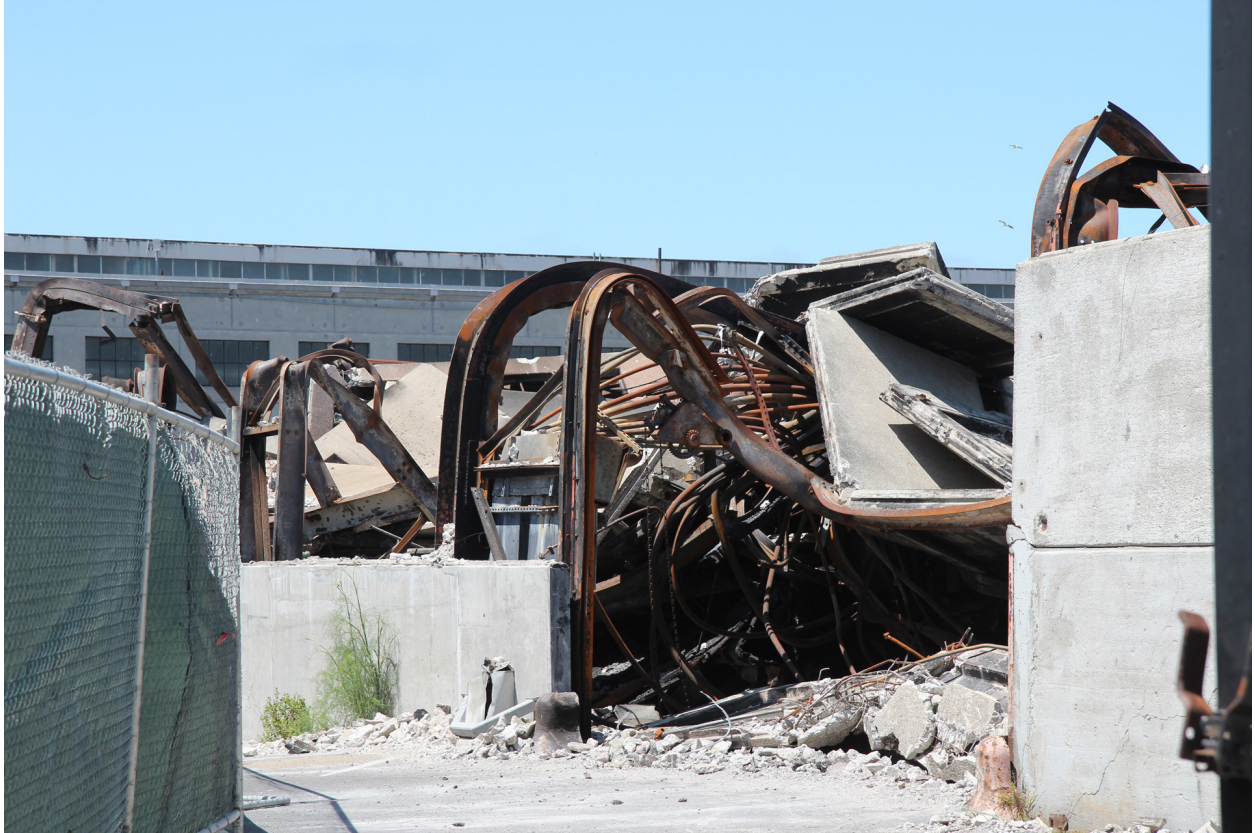
Figure A.3: Failure of south-side perimeter columns as seen from the area between Shed A and Shed C.
