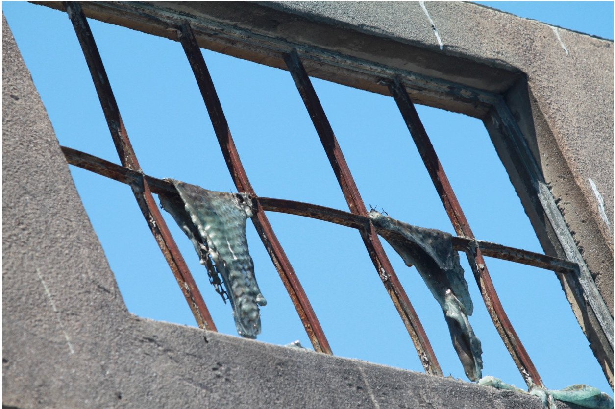
Figure 4.20: Molten glass in the east wall.
