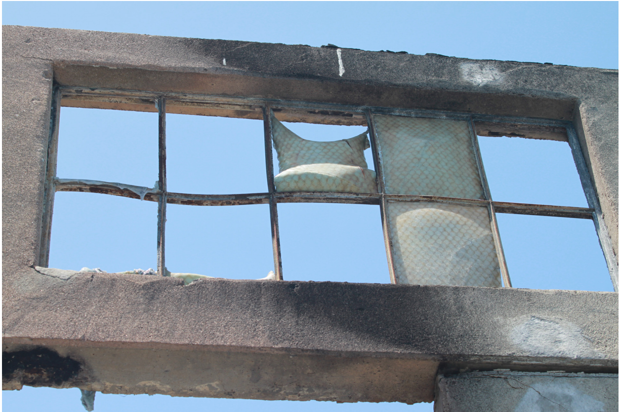
Figure 4.18: Damage to window frame and glass.
