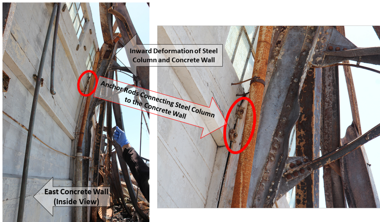
Figure 4.3: Inward deformation of the built-up steel column and concrete wall on the eastern side of the structure.
