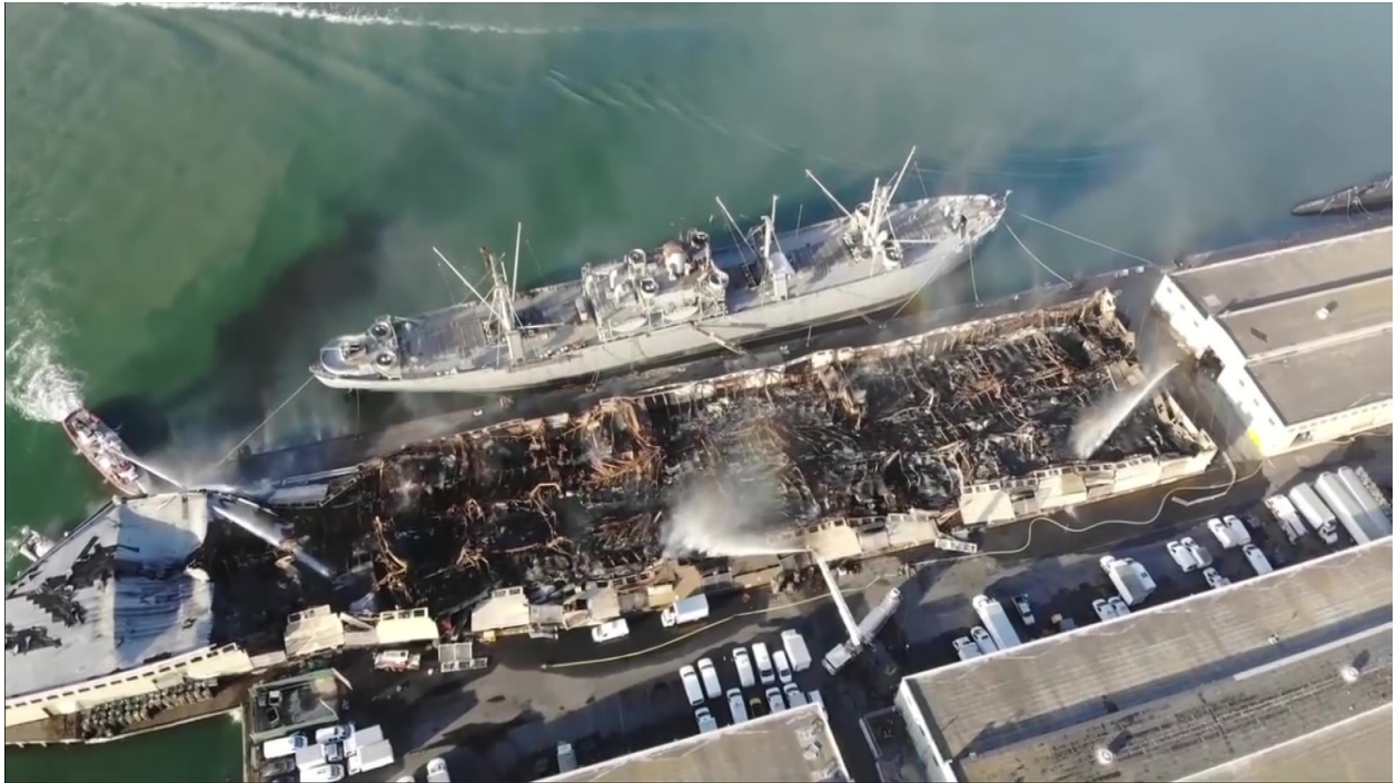
Figure 2.3: Aerial view of Pier 45 showing extend of damage following the fire exposure. (Credit: CBS SF Bay Area, Nathan Wilde)
