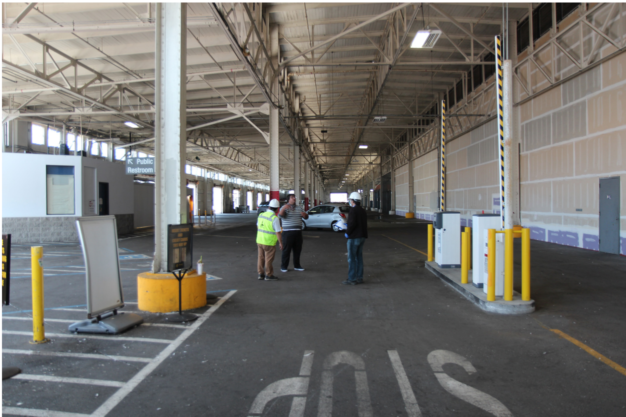
Figure 3.10: This photograph of the passageway in Shed A shows the general structural system in Shed C prior to fire exposure, i.e., the primary structural framing including columns, roof trusses, and W-shaped beams.
