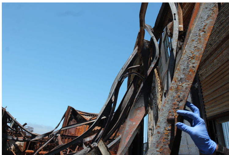
Figure 4.16: Mill-scale peeling on the flange of channel-section beams.
