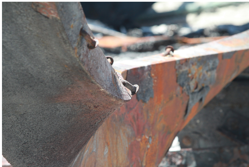
Figure 4.11: Close-up view of out-of-plane deformations in the beam from thermal gradients and restrained thermal expansion.
