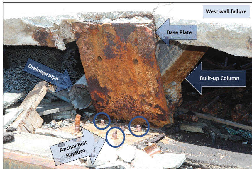
Figure 4.9: Typical pull-out and failure mechanism in the anchor bolts in the west wall.
