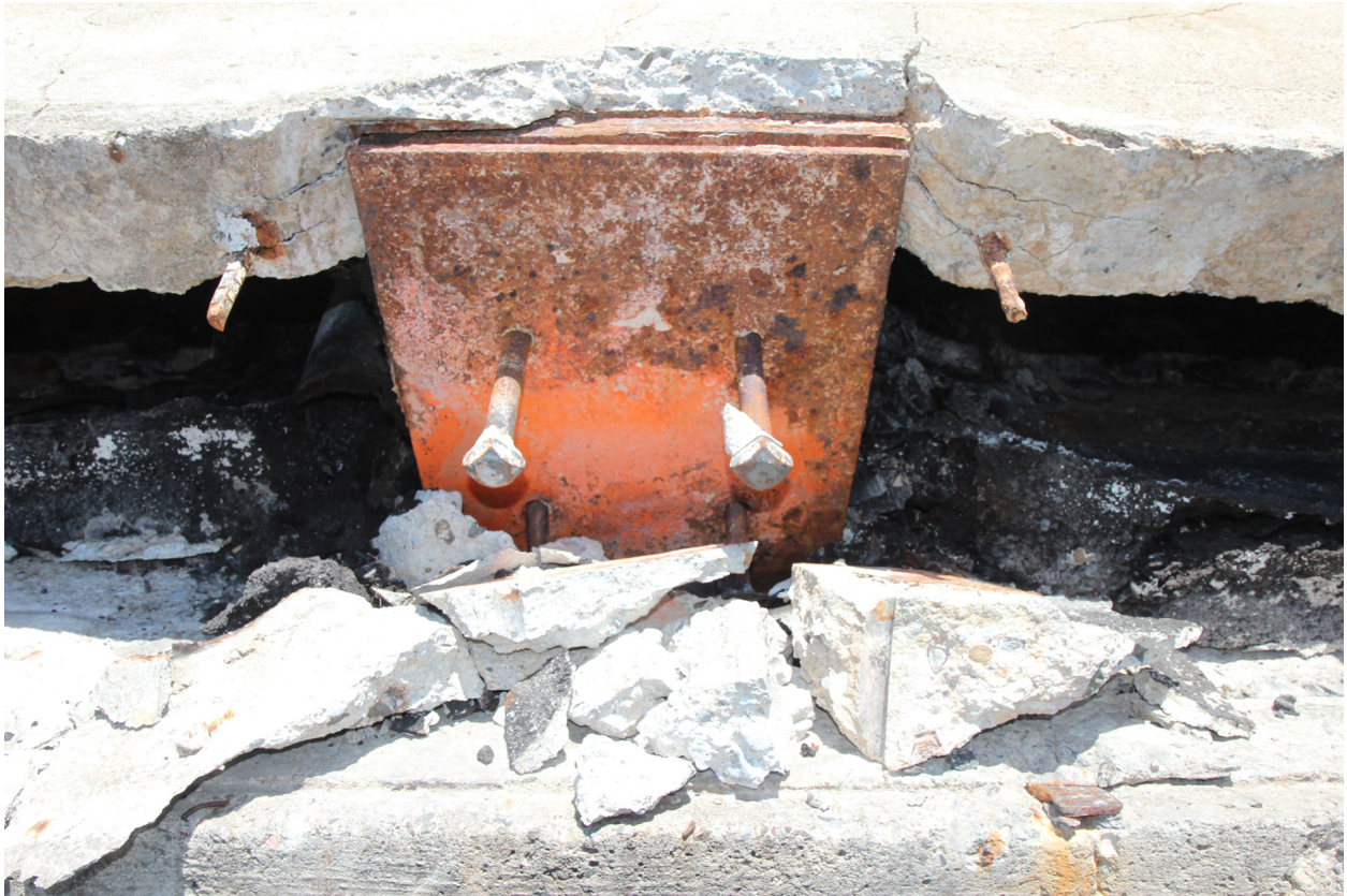
Figure A.4: Anchor bolt pull out in west wall.
