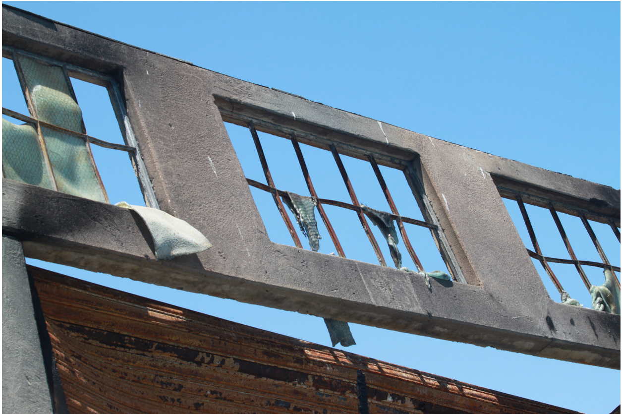
Figure 4.19: Damage to window frame and molten glass in the east wall.
