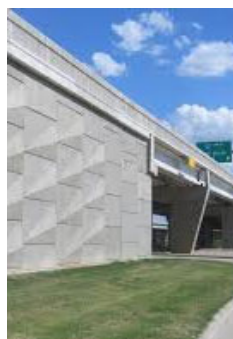
MSE Bridge Abutments
