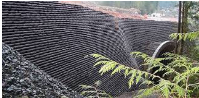
Mechanically-stabilized earth walls
