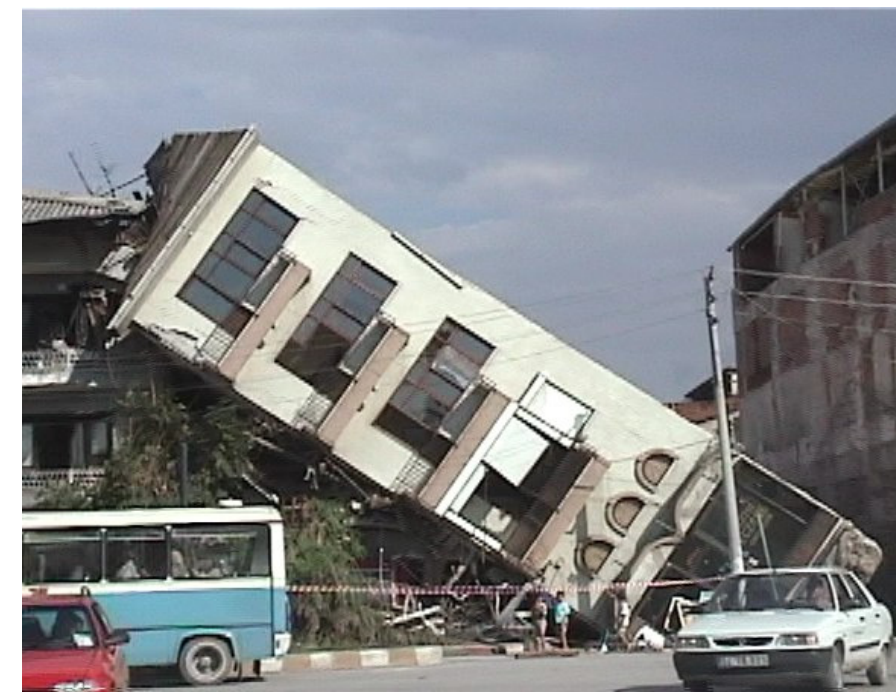
Ground failure in silt, Adapazari 1999
