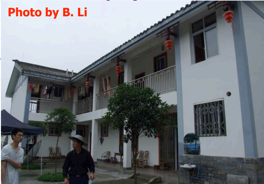
2 story confined masonry residential buildings built in 2006 performed well (Gao Yuan Village)
