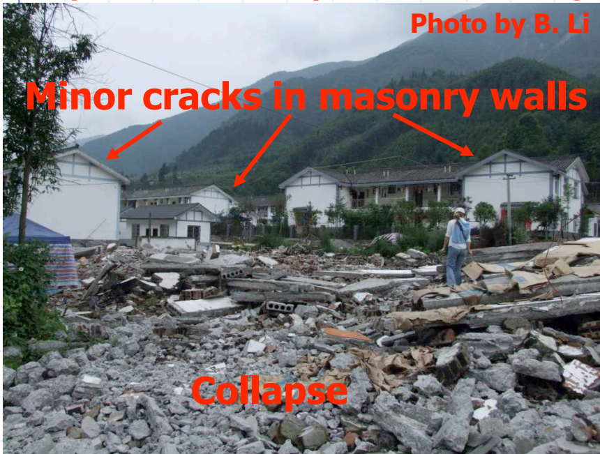
2 story confined masonry residential buildings built in 2006 performed well (Gao Yuan Village)
