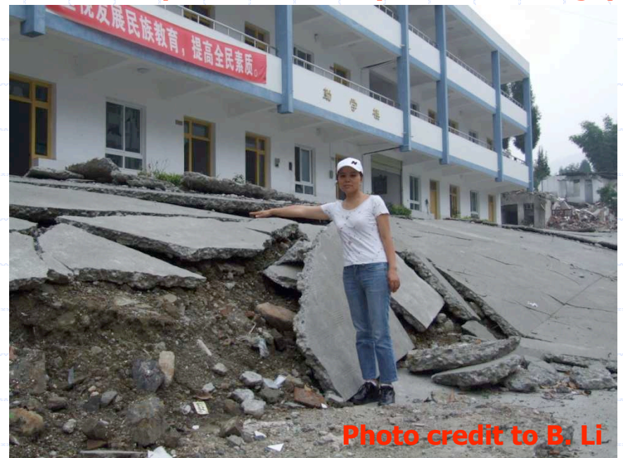
2 story confined masonry residential buildings built in 2006 performed well (Gao Yuan Village)
