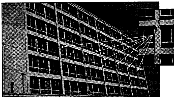
Figure 1. Building frame with column shear failures
