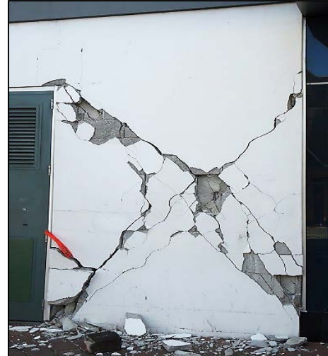
RM damage after the 2011 Christchurch Earthquake
