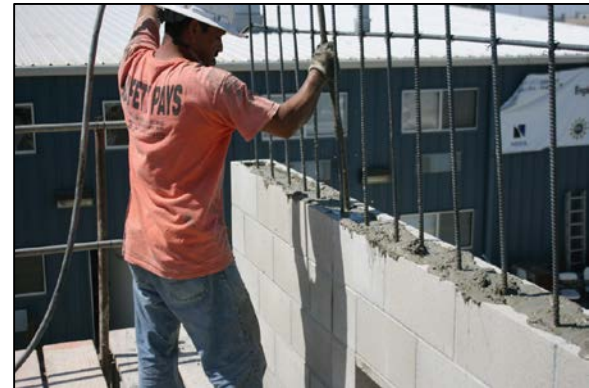
RM wall grouting
