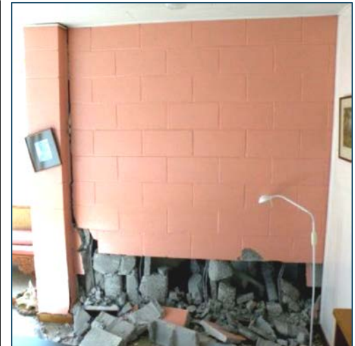
RM damage after the 2011 Christchurch Earthquake
