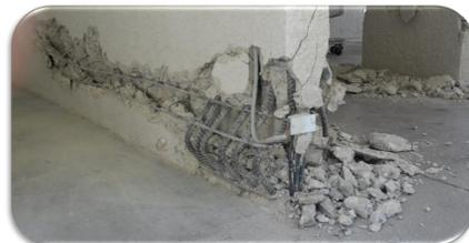
Figure 1. Wall failure after 2010 Chile Earthquake
