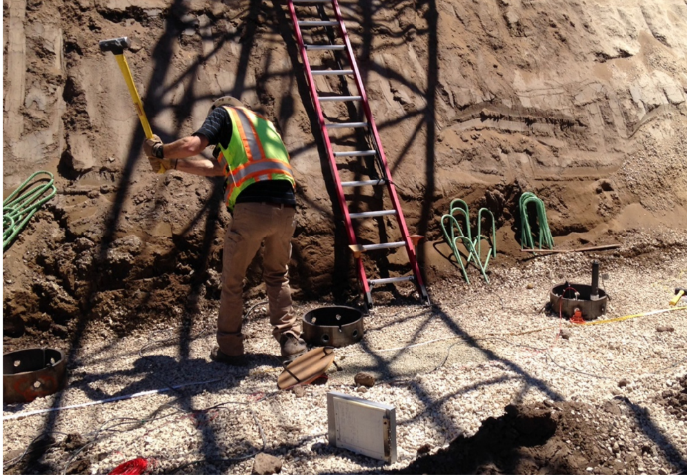
Figure B.4 Striking pile adjacent to test pile.
