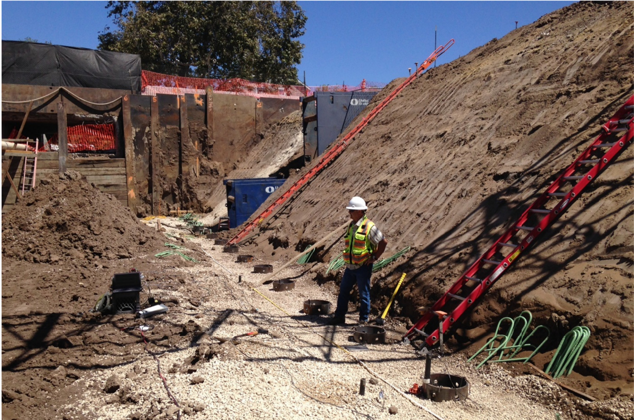
Figure B.2 Pilot study test site.
