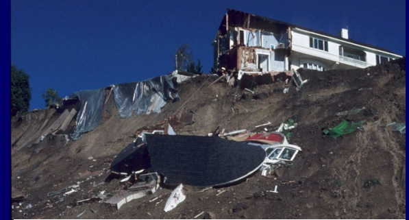
Pacific Palisades Slope Failure
