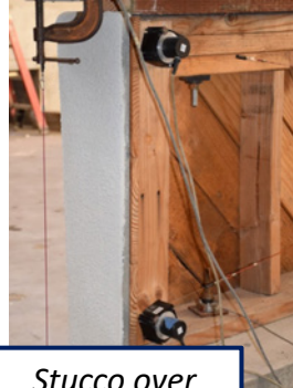
Stucco over diagonal sheathing
