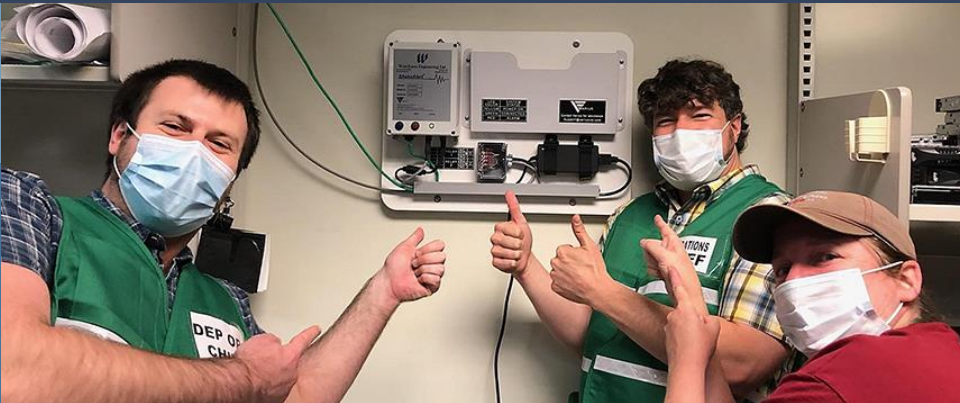
EEW Equipment: Installation & Periodic Replacement
