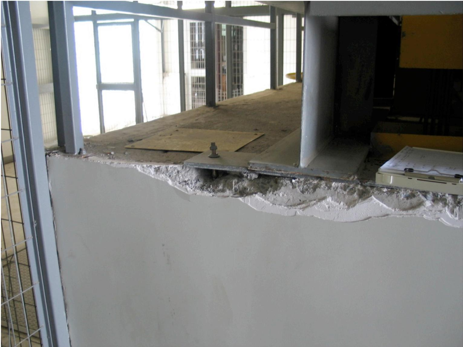
Anchor bolt failure of elevator generator set due to inadequate edge distance.
