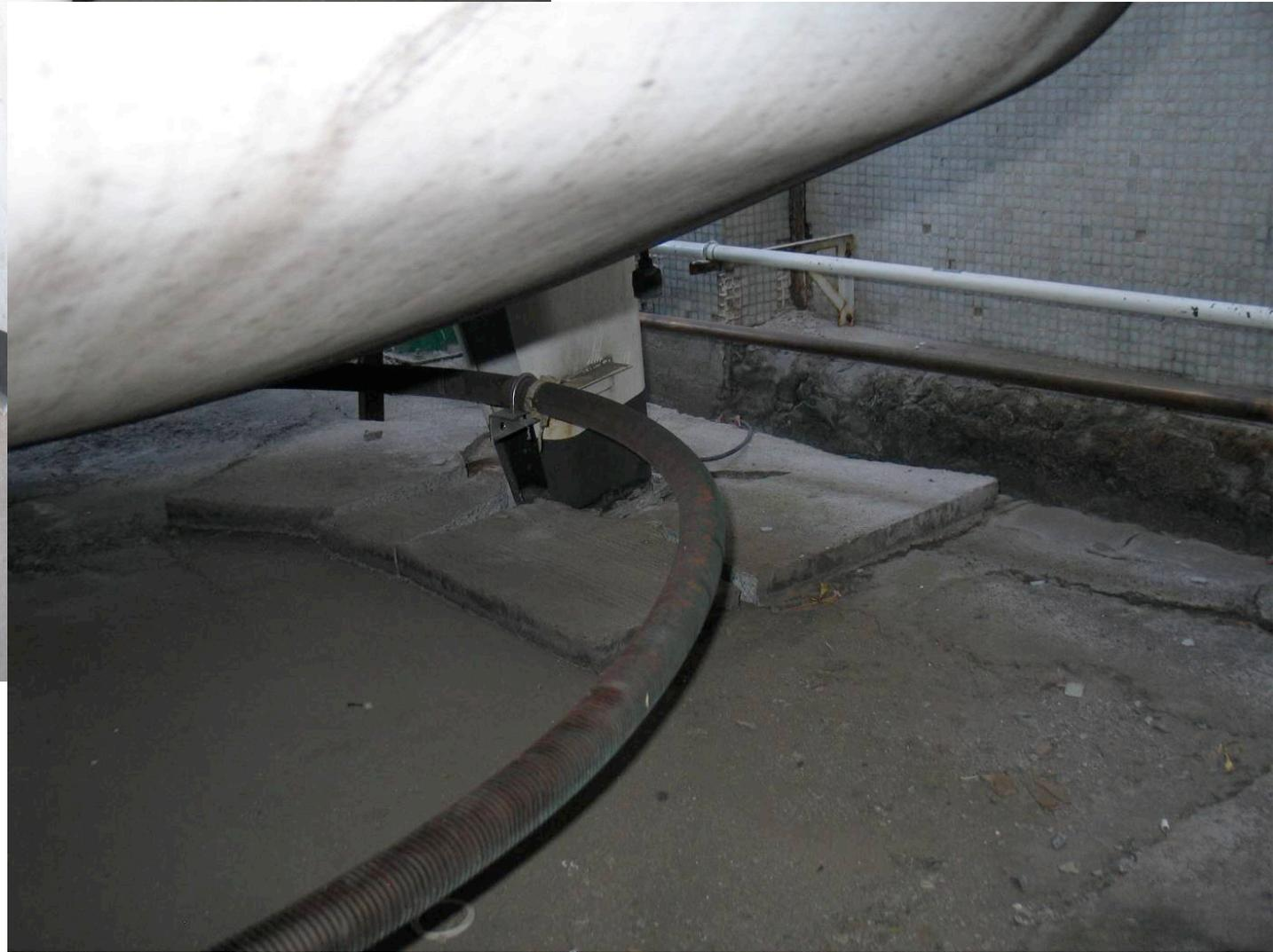
Oxygen tank legs punched through support slab but did not overturn and remained functional.
