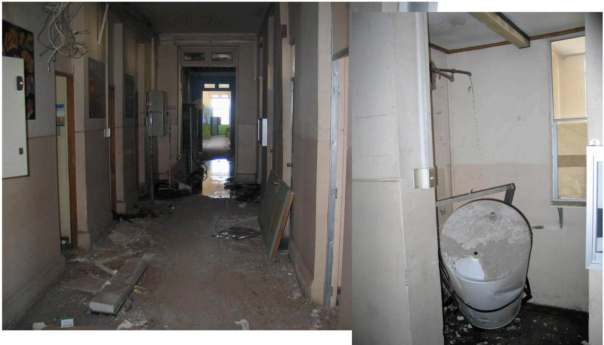
Continuing water damage at Talca Hospital. Water is leaking from water heater on right. Building was closed due to nonstructural damage, dominated by water.
