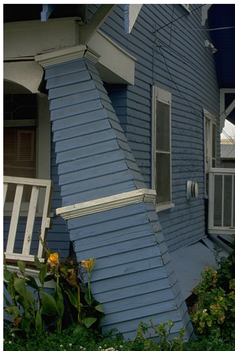
A close up of a collapse-free house in Santa Monica that was none-the-less damaged heavily by the 1994 Northridge Earthquake. "Northridge Earthquake, California". Photograph. 1994. Photograph by FEMA News Photo taken on 01/17/1994 in California. Federal Emergency Management Agency. 20 Sept 2013.
