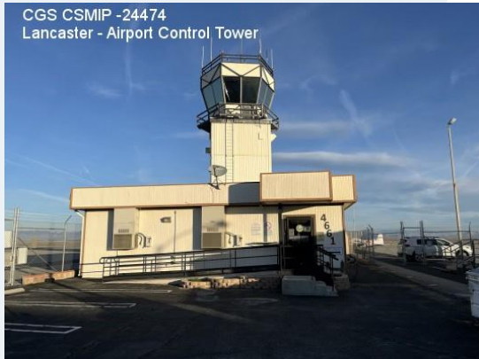
Lancaster Airport Control Tower CSMIP Station #24474
