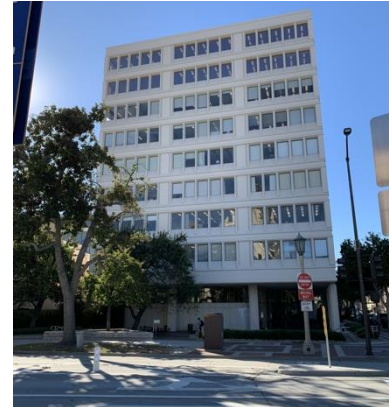
Pasadena – Mutual Savings Bldg. CSMIP Station #24571
