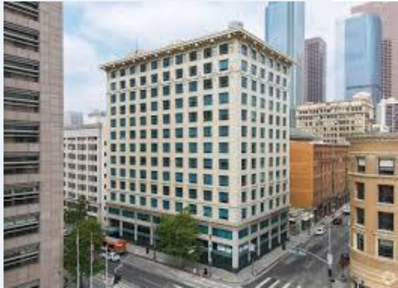
Los Angeles – 311 S. Spring Street CSMIP Station #24567
