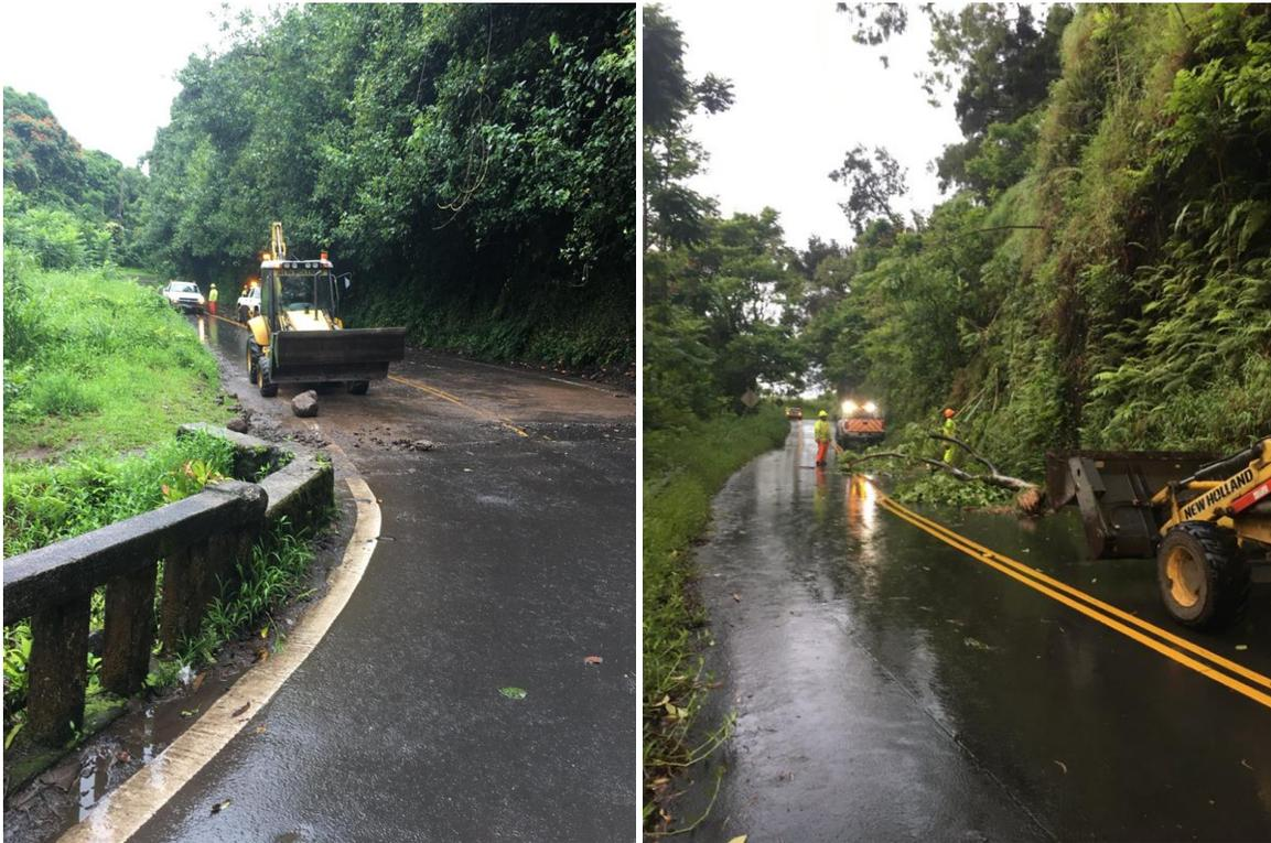
Figure 14: County crews clearing rockfalls and downed trees on Hana Highway, Maui. (Photo Credit: HDOT Twitter Feed – 8 AM and 8:30AM 8/23)
