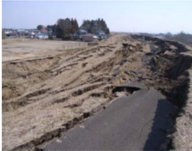
Figure 1. Damaged levee of the Naruse river
