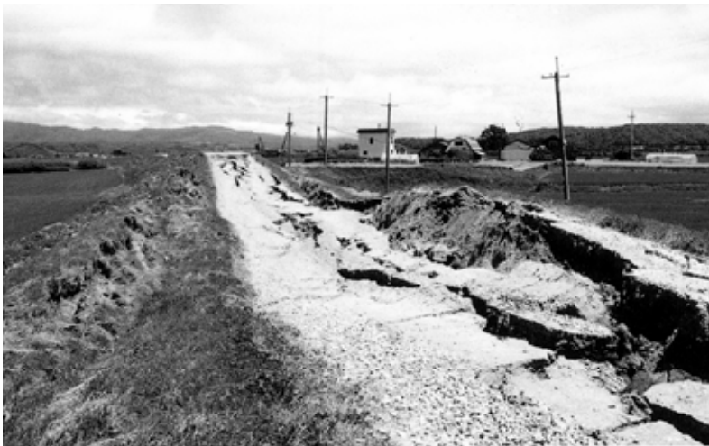
Figure 1. Damage to a river dike at the Shiribeshi-Toshibetsu river, Hokkaido, Japan, during Hokkaido-Nansei-oki earthquake of 1993 (Iai and Ichii, 2010)
