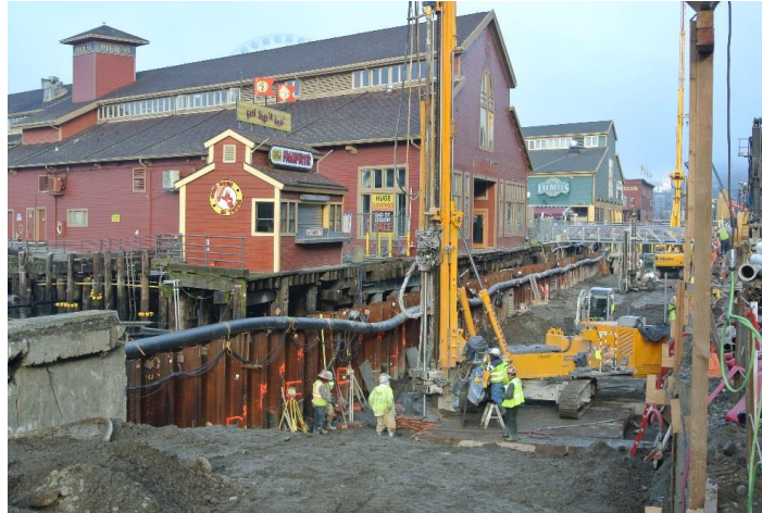
Figure 6.2 Jet grouting of cellular wall structure adjacent to sensitive historic piers along Seattle waterfront ( http://sdotblog.seattle.gov ).
