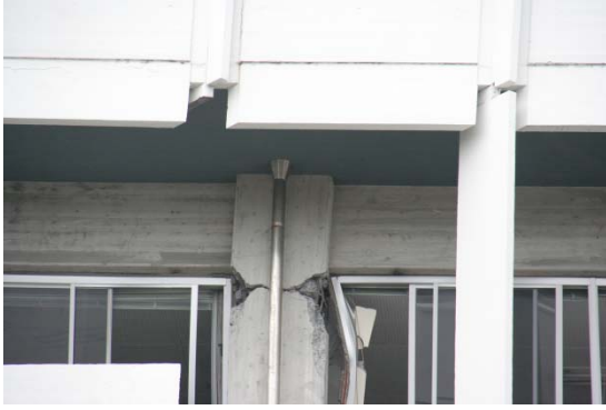
Flexural failure at the top of an interior column in fifth story
