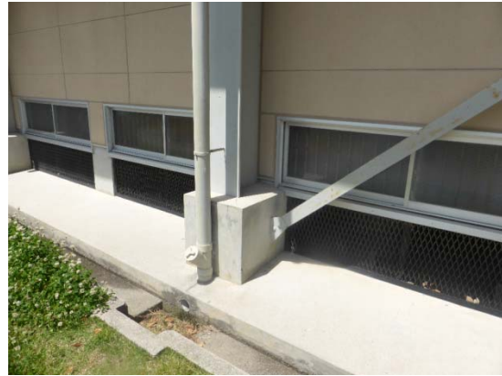
Cracking in a concrete foundation of the brace
