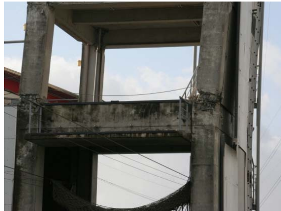
Flexural failure at the base of third story columns
