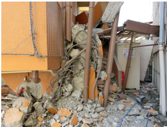
Collapsed column at the northeast corner
