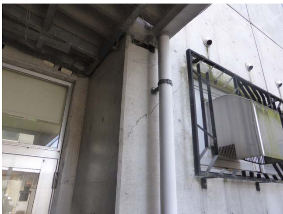
Shear cracks on a short column
