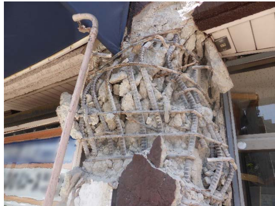
Shear failure at the lapping of reinforcement
