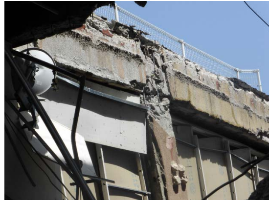
Failure of a beam-column joint at the top of a second story column
