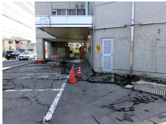
Broken asphalt around the building
