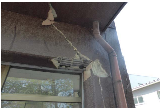
Shear failure of a beam
