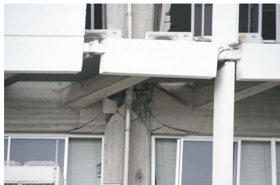
Failure of an interior beam-column joint at fifth floor on south side of the building
