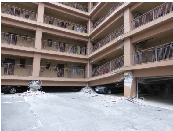
Soft 1 st story collapse in north east frame
