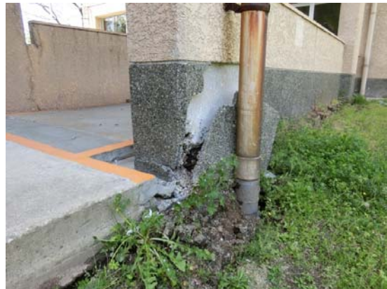
Damaged column of the corridor
