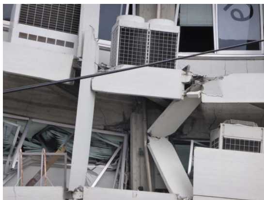
Failure of an interior beam-column joint at the fifth floor on west side of the building
