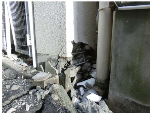
Damage to the column of the connecting corridor
