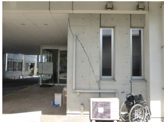
Shear cracks in the nonstructural panel (due to subsidence of the supporting ground)
