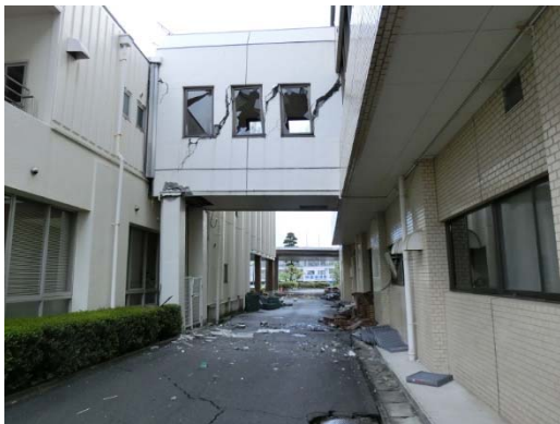
Damaged connecting corridor
