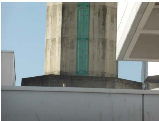
No damage at the bottom of the chimney
