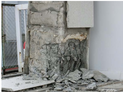
Damage to corner column
