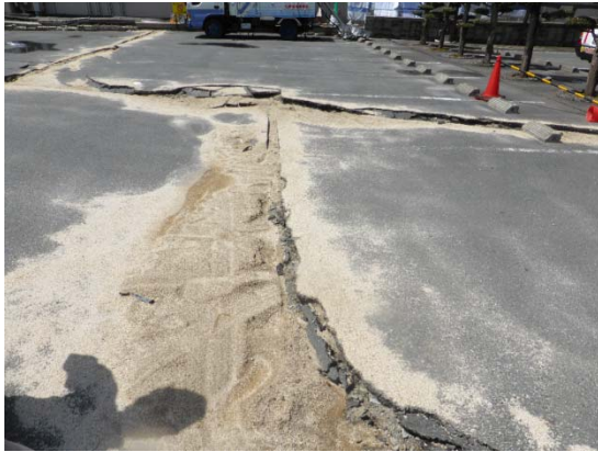
Ground opening in the parking
