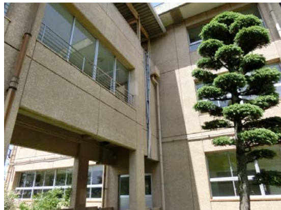
Displacement at the expansion joint between the corridor and the school building
