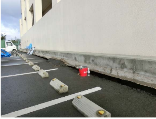
Settlement around the outer frame
