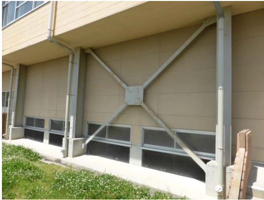
Steel braces in the first story of the gymnasium
