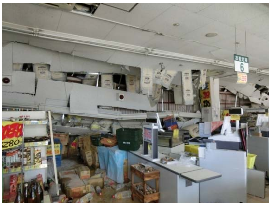
View of the damage from inside the building in the first floor. (The upper floor collapsed down)
