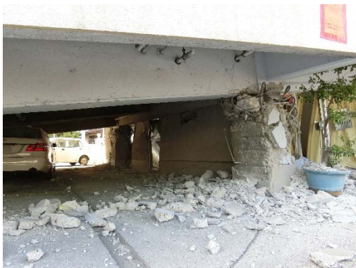
Axially crushed north columns
