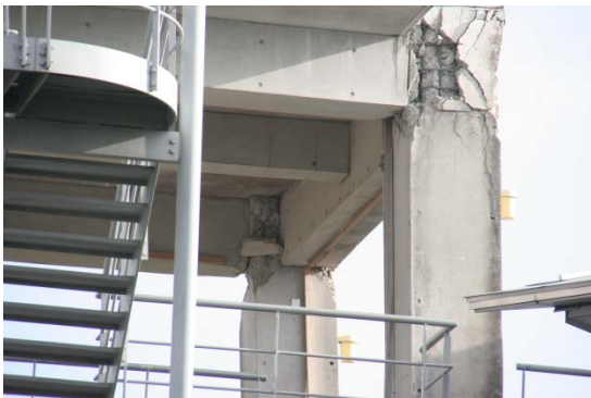
Failure in the beam-column joint at fourth floor
