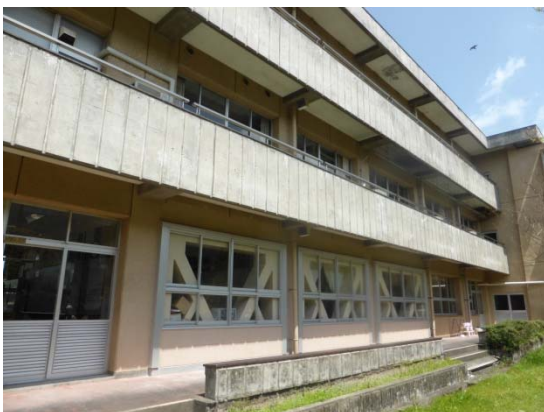
Seismic retrofitting by steel-braced frames
