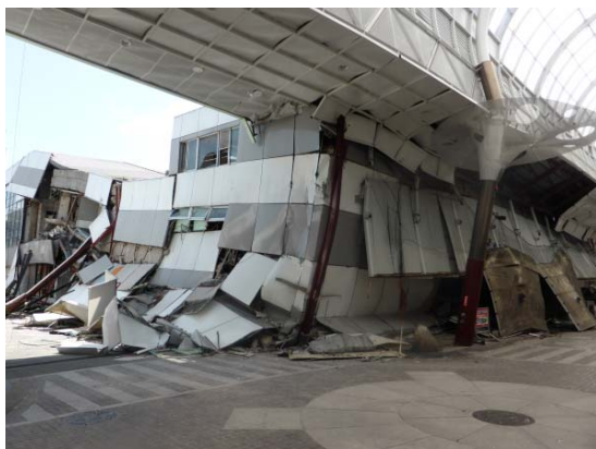
Building leaning against the columns of the arcade
