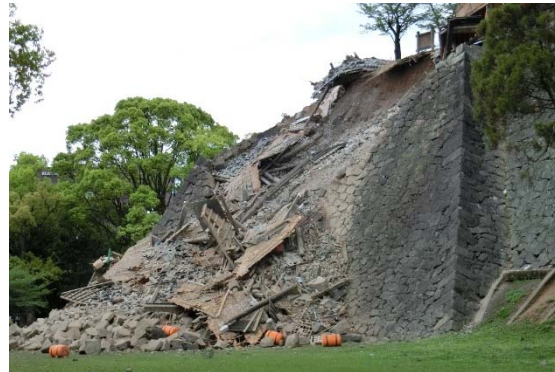
Collapsed Higasi-Jyuhakken turret and the surrounding stone retaining wall
