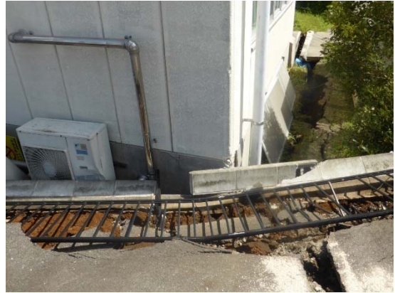
Ground displacement at the back of the building
