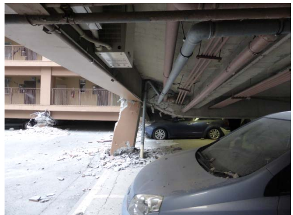
Bending of the transverse beam in north frame
