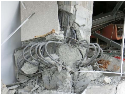
Axially crushed column
