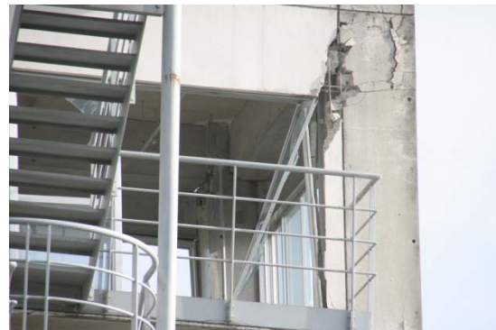
Failure in the beam-column joint at fifth floor
