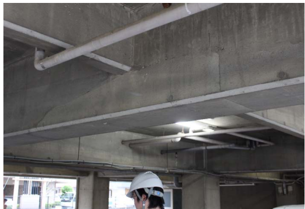
Vertical cracks at the middle span of a beam
