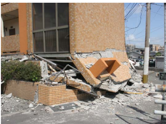
Failure of the gable wall at the south side
