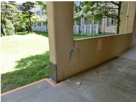
Cracks at the end of spandrel wall in the corridor
