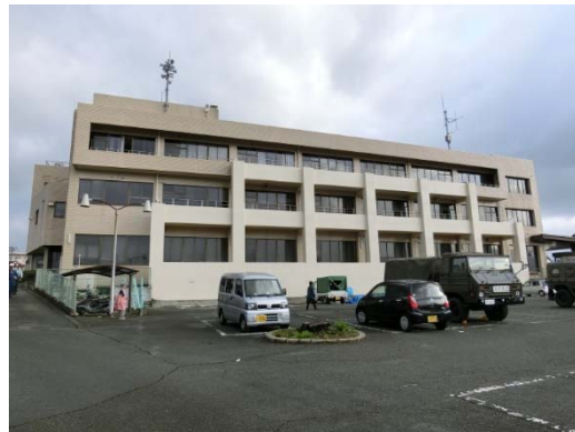
South view (retrofitted with an outer frame)
