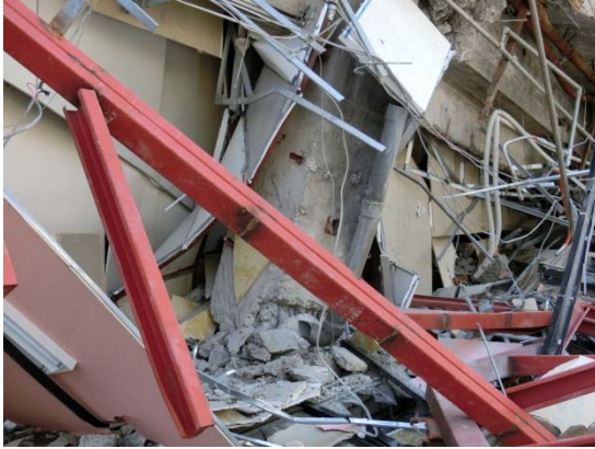
Collapsed column in the first story
