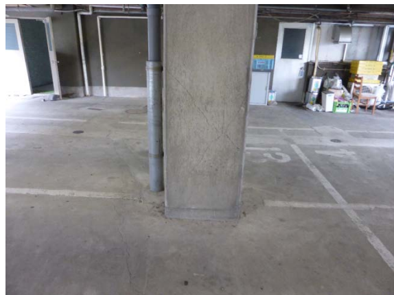
Shear cracks in a first story column
