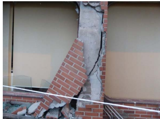
Shear failure in a column
