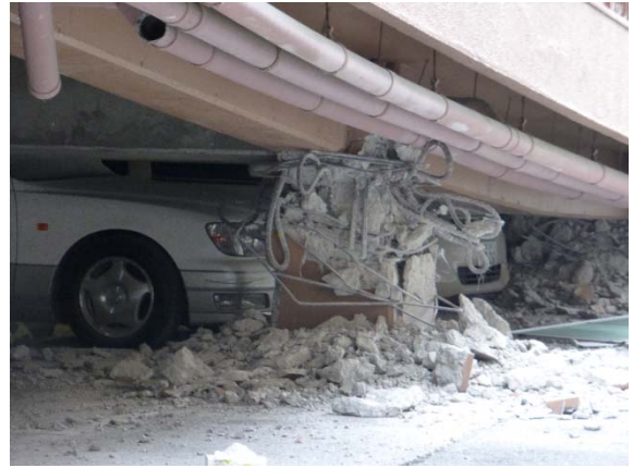
Crushed column in the south frame
