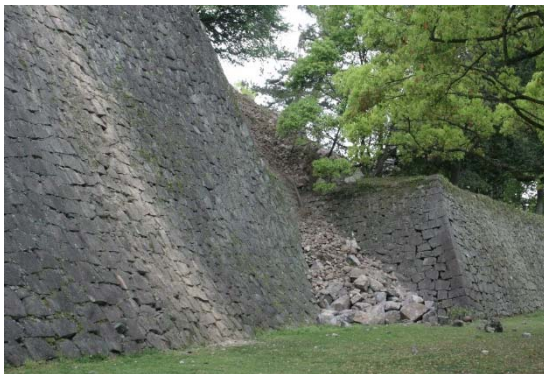
Collapsed Kita-Jyuhakken turret and the surrounding stone retaining wall
