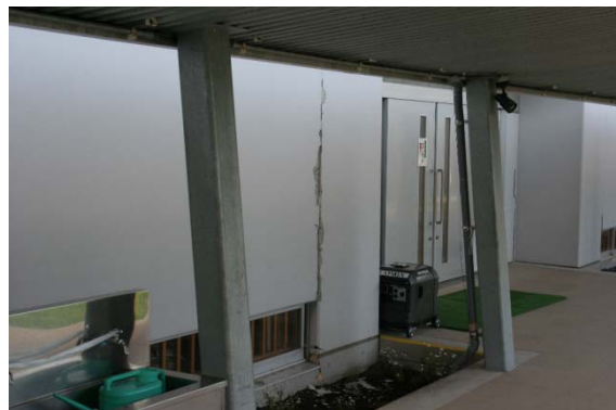
Damage to the exterior walls
