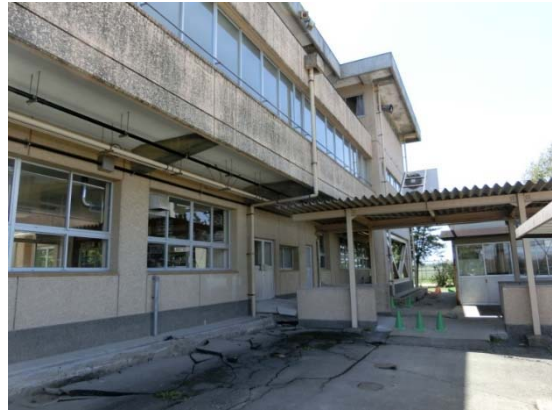
Ground displacement around the school building
