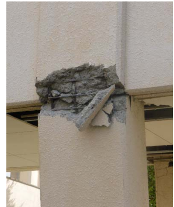
Top of the damaged column (connecting corridor)
