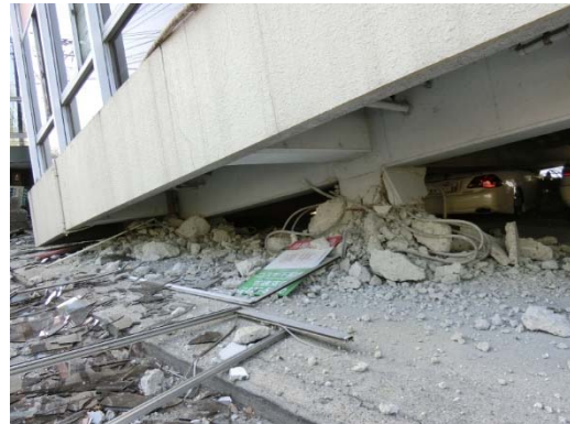
Axially crushed south columns
