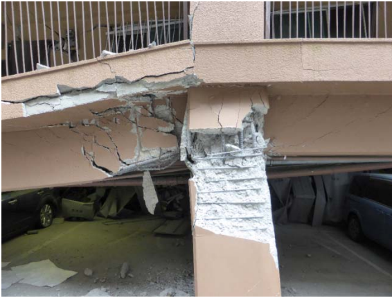
Column damage in the north frame
