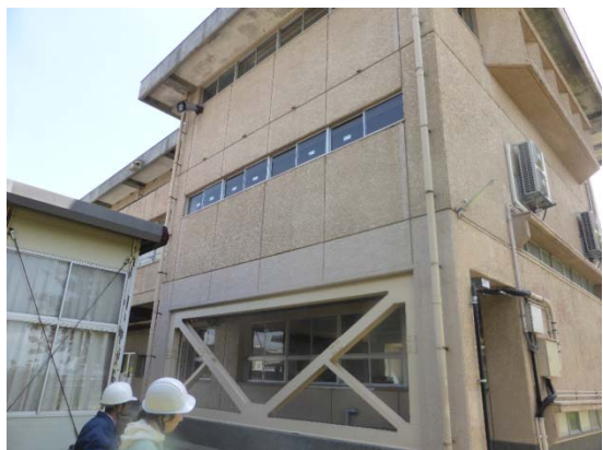
Seismic retrofitting by steel-braced frames
