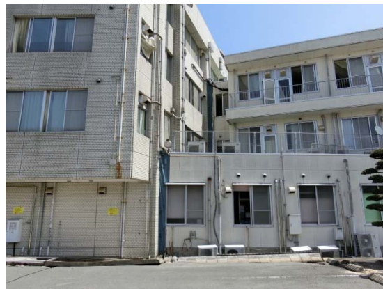
Displacement across the expansion joint
