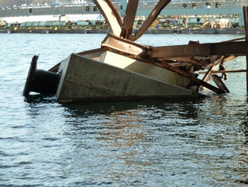
*Damage to pier and warehouse due to multiple impacts from single loose ship*
