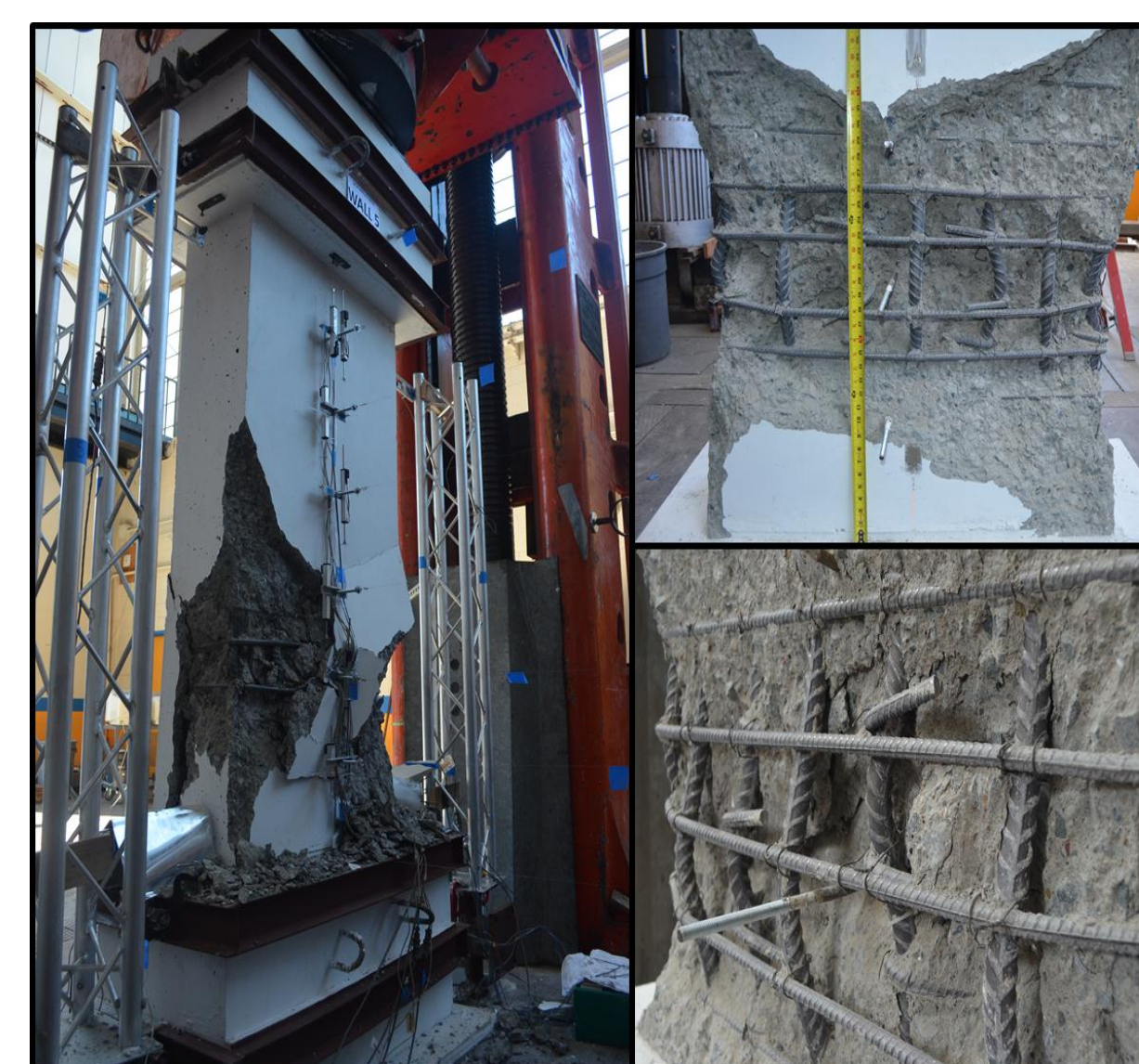
Figure 5. 2013 Wall 5 failure after being tested at NEES Laboratory in Richmond Field Station.
