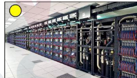
Aurora (scheduled 2024) Argonne National Lab Argonne Leadership Computing Facility (ALCF) 10,624 GPU accelerated nodes 6 Intel Max GPUs / node Projected ~ 2 ExaFlops Undergoing final assembly
