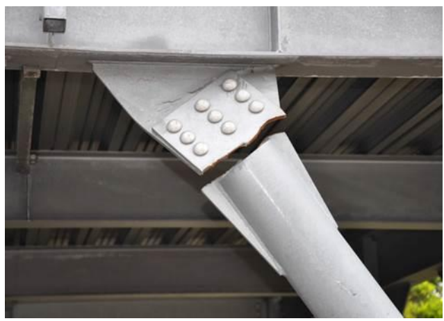
Figure 2: Complete fracture of gusset plate (Lignos, 2011)
