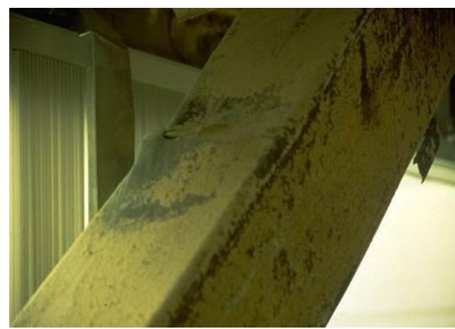
Figure 3: Local buckling of square HSS brace (NISEE, 1994)
