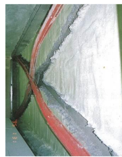
Figure 4: Global buckling of braces (AIJ, 1995)
