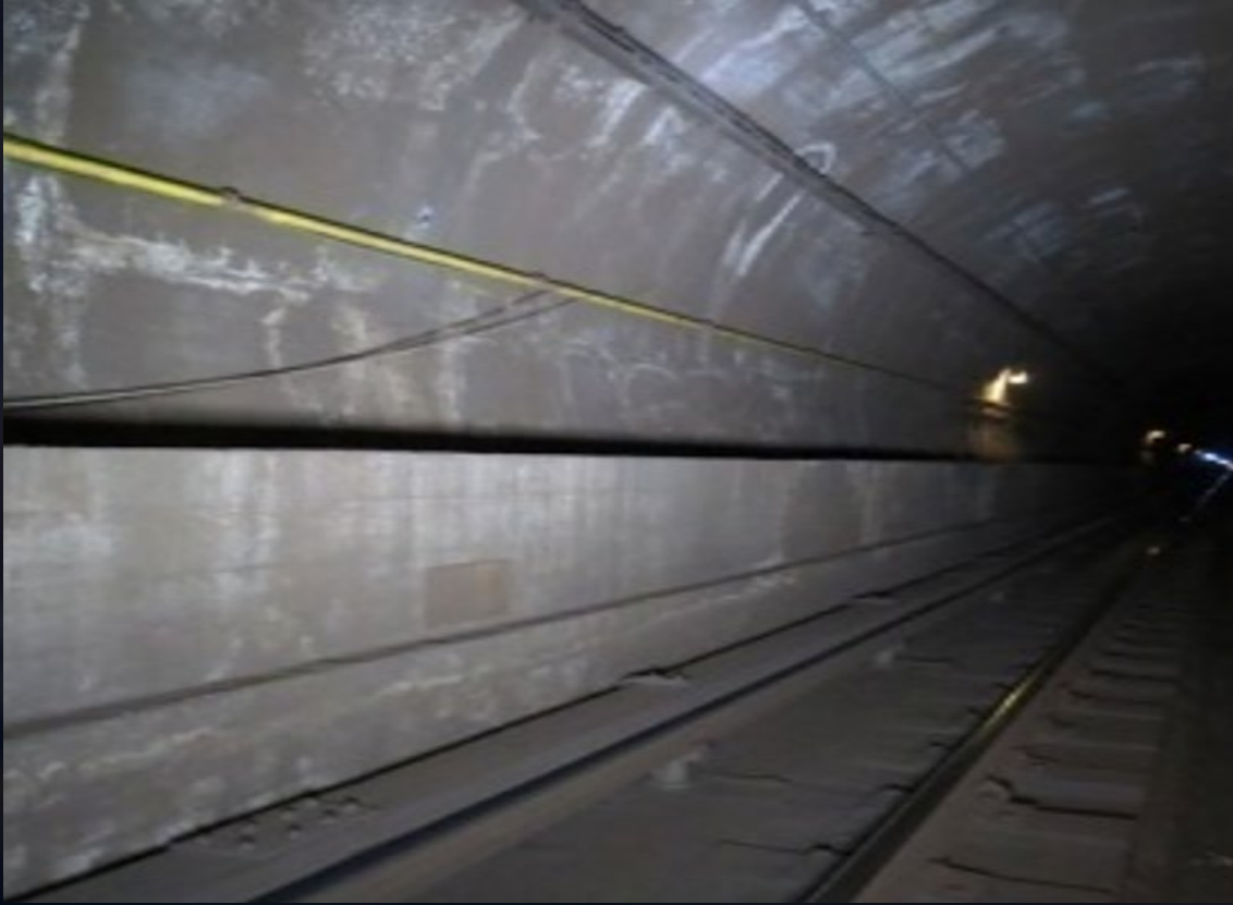
Example of cement benchwall in good condition.
