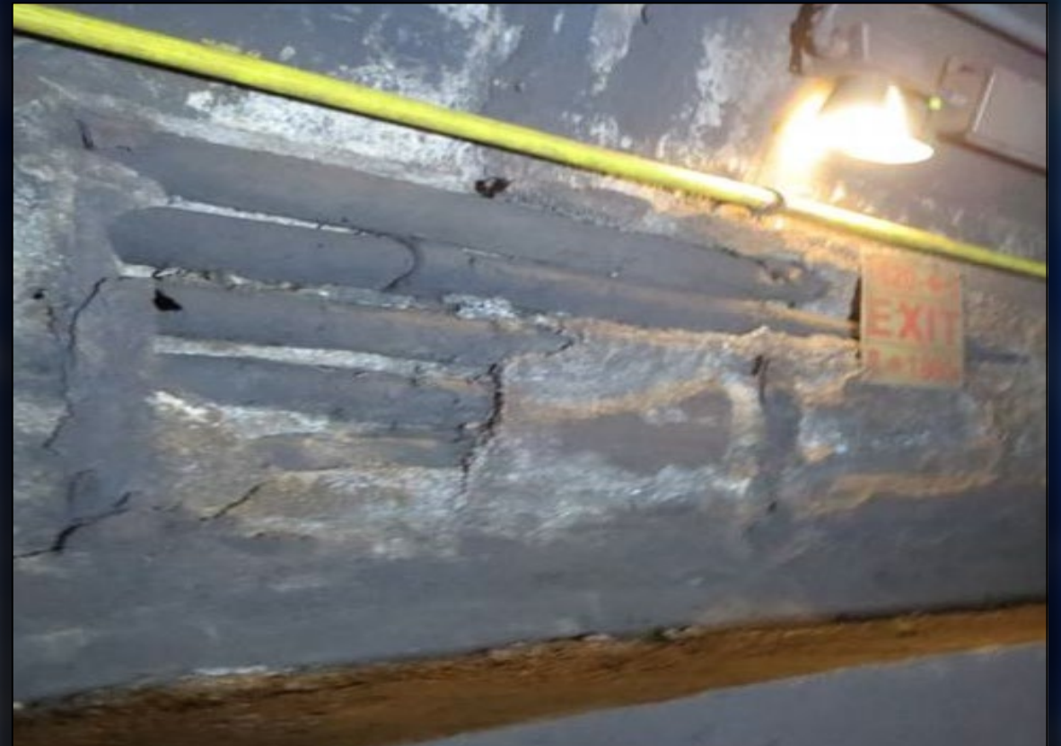
Concrete deterioration: alkali silica reaction
