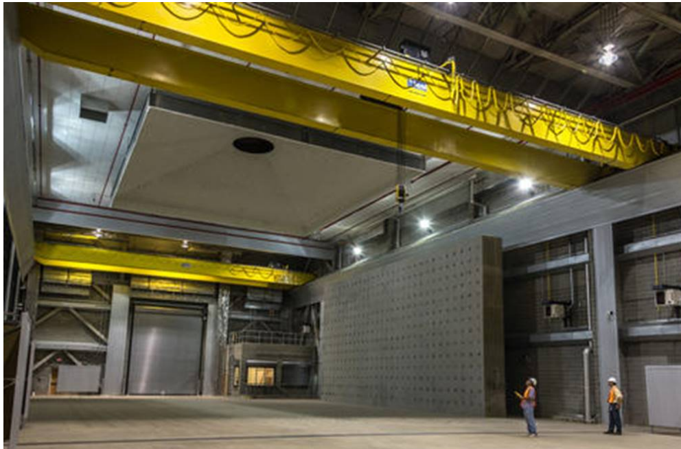
Figure 1: National Fire Research Laboratory at the National Institute of Standards and Technology (source: https://www.nist.gov/el/fire-research-division-73300/national-fire-research-laboratory-73306 )
