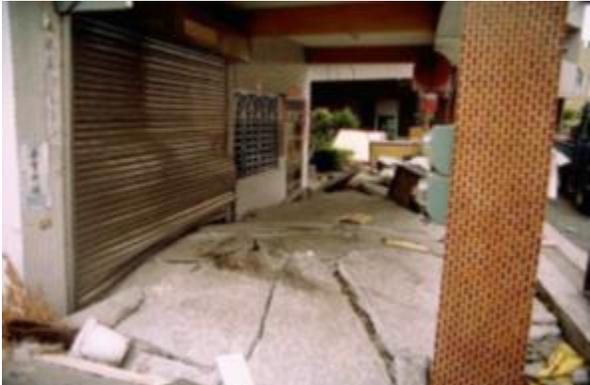
**Figure 1.2** Typical foundation failure (punched footings and intermediate slab heaving). (Chu et al. 2008). Photo by R. Seed (1999)
