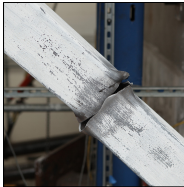
Figure 5.5 Final fracture state of the west brace.
