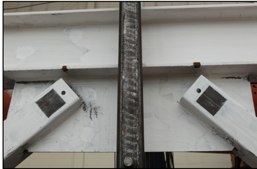
Figure 5.11 Center gusset plate at the roof.
