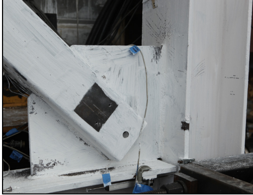
Figure 5.10 West gusset plate at the second story.
