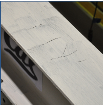
Figure 5.17 Top of roof beam above the center gusset.
