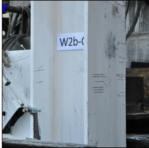
Figure 5.7 Base of west column at second story.
