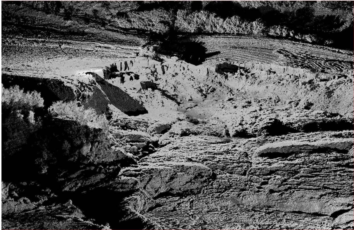
Figure 3.7 Detailed LIDAR of head scarp of Las Palmas tailings dam failure (from GEER [2010]).
