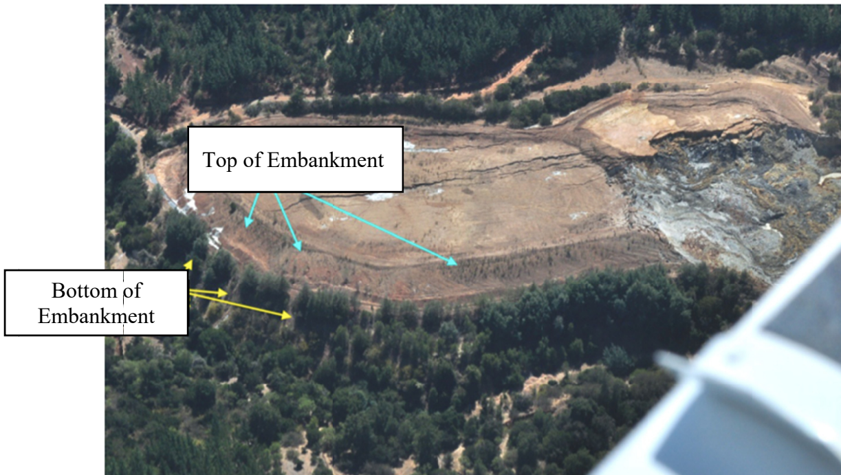
Figure 3.3 Aerial photograph showing scarp, longitudinal cracks, and the location of the tailings dams (after DICTUC [2012] and Gebhart [2016]).
